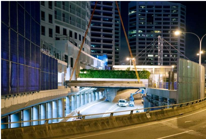
Figure 14 Night works at the 161 Sussex Street development. Multiplex has experience craning precast beams into position over the Western Distributor.
