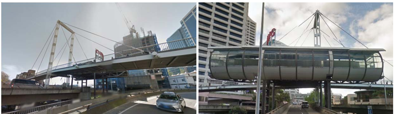
Figure 8 Cable-stayed bridge linking Pymont Bridge with Sussex Street and Existing Monorail Station. Aerial view. (Google Maps, 2017)
