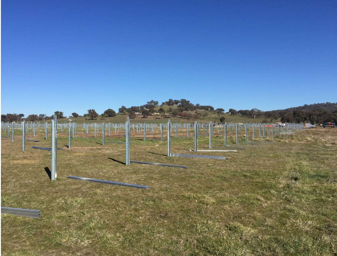
a) Tracking piles, during construction.
