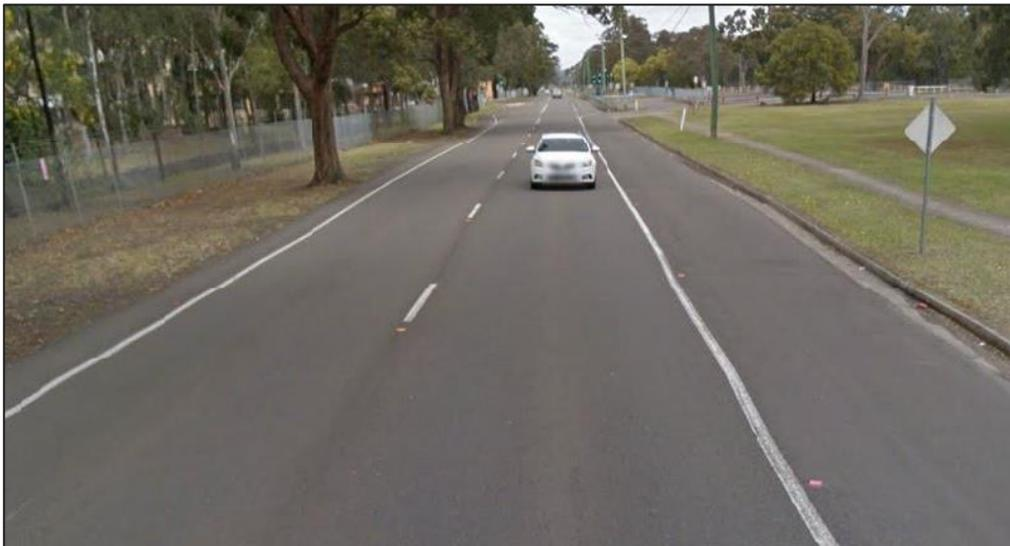
**Figure 2-8 Sealed & marked road shoulders on Moorebank Avenue – permitted for on-street cycling**
