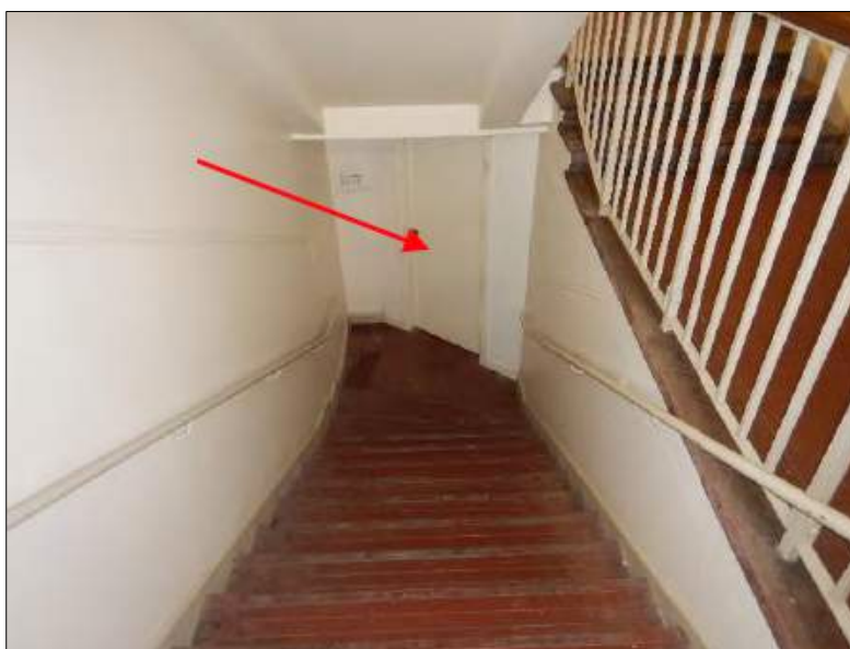
Figure 42: Looking towards the base of the staircase in Building 1B and the storeroom, Room 107 (marked by the arrow). This room has been created with plaster board walls. It has a plaster board ceiling and flush panel door. CMP 2016.
