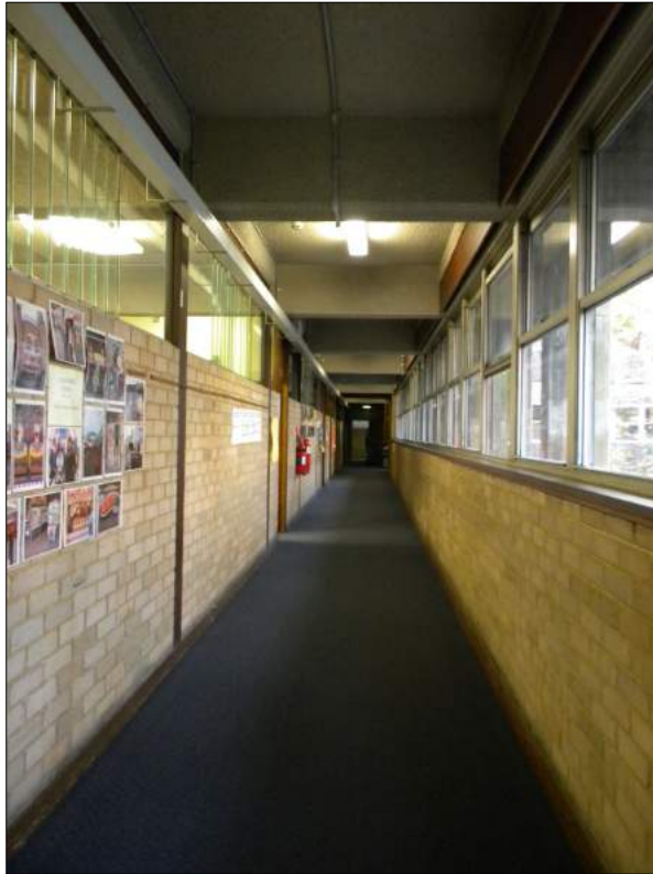
Figure 135: Typical corridor within Building 4 with face brick walls and coffered vermiculate ceiling. The interior walls of classrooms/staffrooms have glazing to the top. Doors are single panel doors.
