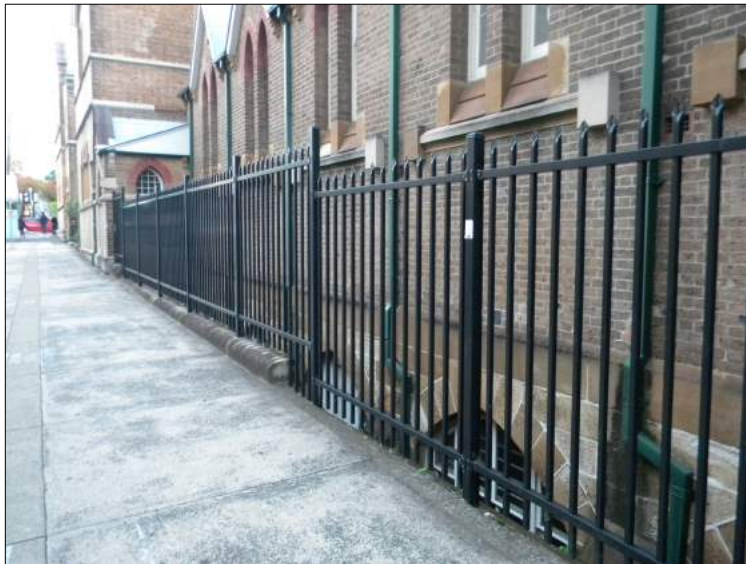
Figure 12: Modern steel palisade fence, part of which is set into a stone base outside Building 1 on Chalmers Street.
