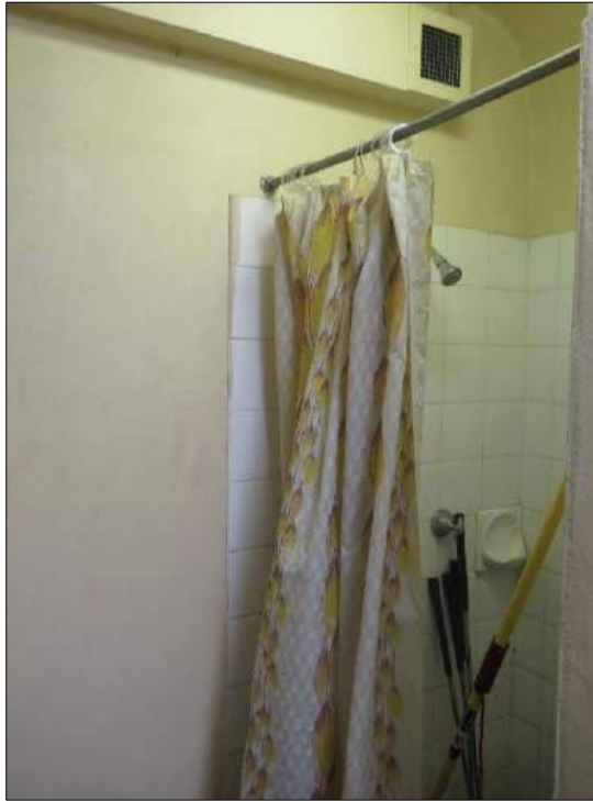
Figure 43: Room 115 in the CMP 2016 . The walls are of rendered masonry, with later tiles. The ceiling, cornice and skirting are of concrete.
