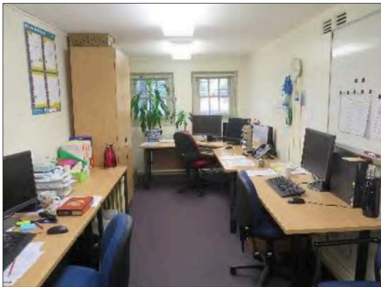
Figure 49: Room 131 in the CMP 2016 . This room has rendered walls and a concrete ceiling; timber skirting boards and architraves. The door from the hallway is a modern flush door. CMP 2016 .
