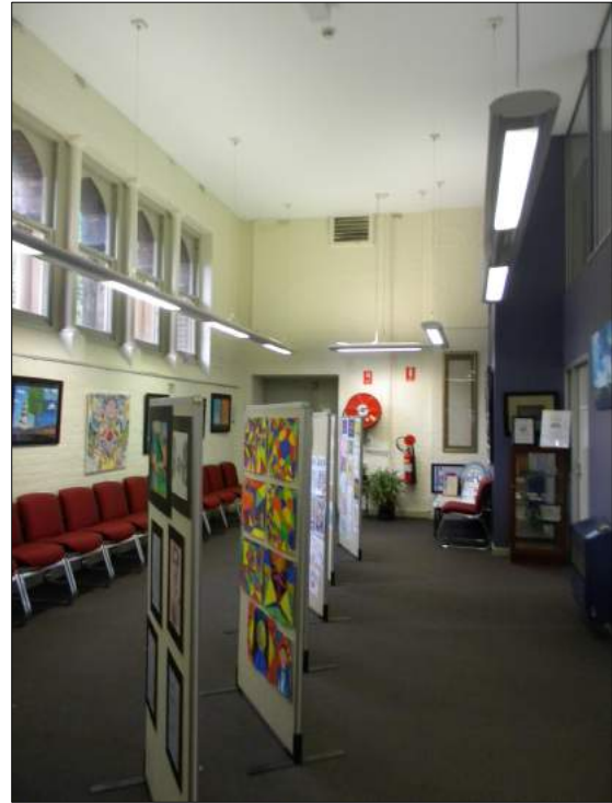
Figure 98: Room 205 in the CMP 2016. Original walls are of painted brick or are covered in plasterboard. There are modern partitions and a later plasterboard ceiling within this space.
