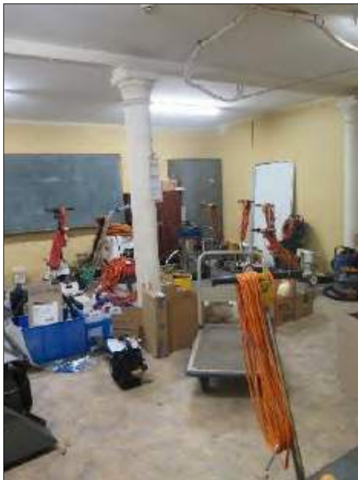
Figure 38: Room 101. This room, and Room 102, have rendered and painted masonry walls and plasterboard ceilings. It is not clear what lies beneath the modern floor coverings. The CMP 2016 suggests that there may be stone flagging. Note the cast iron columns. Doors have been replaced.
