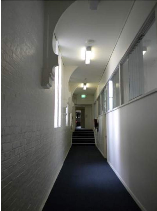
Figure 100: CMP 2016 Room 217. Original walls are of painted brick. The original ceiling is concealed by a later plaster board ceiling. A later partition wall creates the passageway, leading up to the walkway to Building 4.
