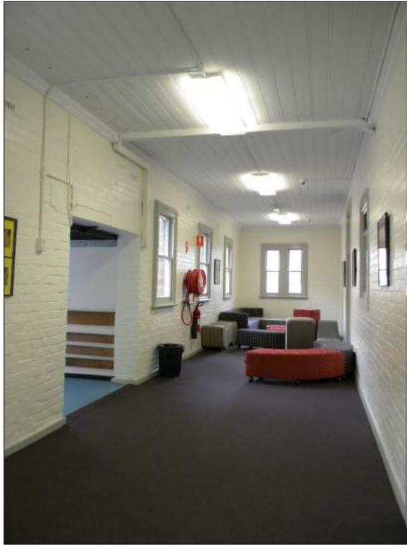
Figure 56: Room 159 in the CMP 2016. This room has painted brickwork walls and a timber lined ceiling. Figure 57: Detail of the opening in Figure 53 leading onto the walkway leading to Building 2B.
