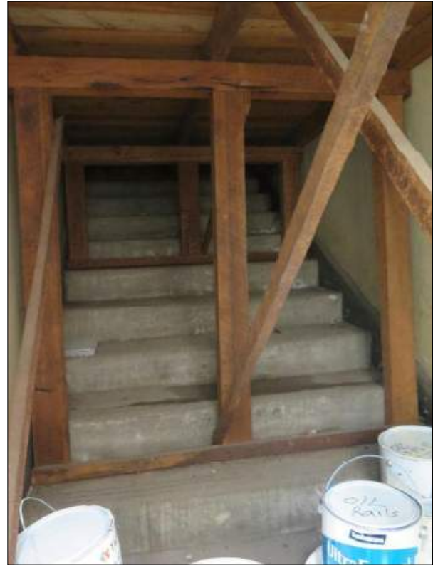
Figure 117: Storeroom beside the staircase (CMP 2016 Room 314). This space has a concrete floor and ceiling and rendered walls. The sink, just visible, is modern.
