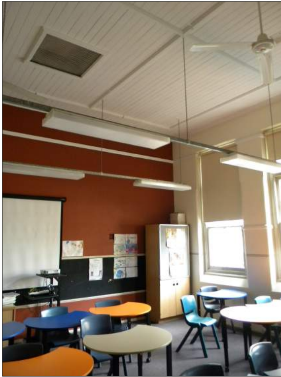
Figure 55: Room 149 in the CMP 2016 . This room has rendered walls and a timber lined ceiling.
