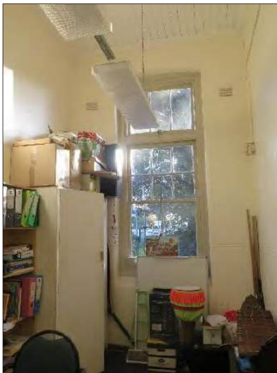
Figure 52: Room 141 in the CMP 2016 . This room has rendered walls with a dado line and rendered skirtings; a timber lined ceiling and timber architraves. The door to the hallway has been replaced.
