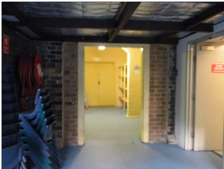
Figure 95: Looking towards the original exterior wall at ground floor level of Building 2A within the walkway. The double doors visible in the distance open into Room 210. They are set in a later plaster board wall.
