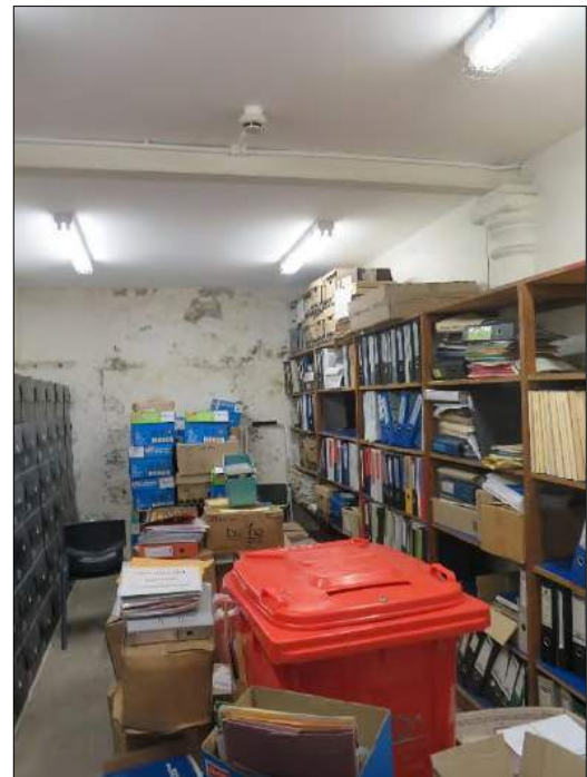
Figure 38: Room 101. This room, and Room 102, have rendered and painted masonry walls and plasterboard ceilings. It is not clear what lies beneath the modern floor coverings. The CMP 2016 suggests that there may be stone flagging. Note the cast iron columns. Doors have been replaced.
