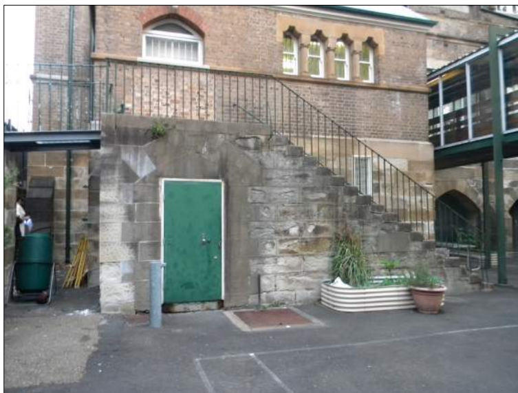
Figure 71: Northern elevation of Building 2A. It is proposed to remove the later infill and door beneath the stairs, reinstate the original opening and install a new door.
