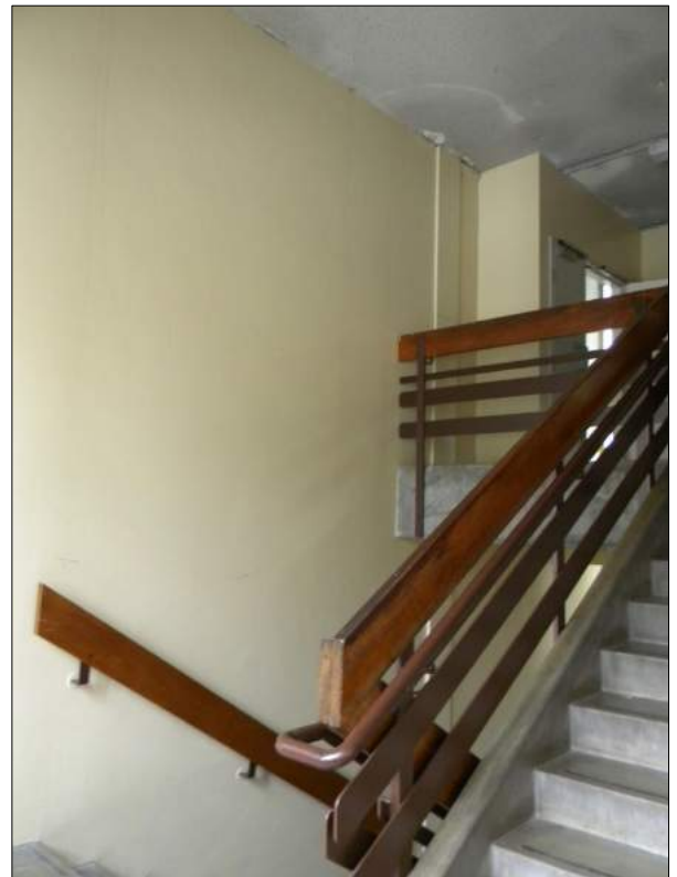
Figure 137: Typical stairwell within building 4, showing concrete stair and timber and metal balustrade.
