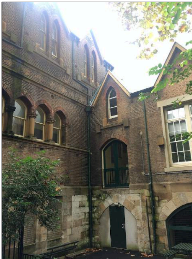
Figures 82 and 83: Western elevation of Building 2A. It is proposed to remove the infill in the lower ground floor opening in Figure 82.
