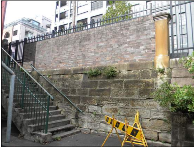
Figure 11: Detail of the stone retaining wall, with brick wall above, adjacent to Building 3 along the Chalmers Street boundary.
