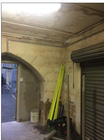
Figure 86: Room 222 in the CMP 2016 . This room has painted masonry walls and a plaster board ceiling. Original openings to either side have been enclosed by roller doors. It is proposed to remove these roller doors.
