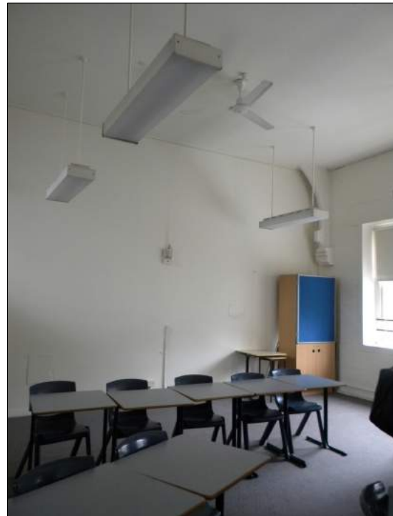
Figure 100: CMP 2016 Room 217. Original walls are of painted brick. The original ceiling is concealed by a later plaster board ceiling. A later partition wall creates the passageway, leading up to the walkway to Building 4.
