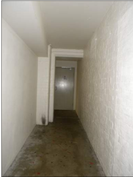
Figure 45: Room 123 in the CMP 2016. This hallway has painted brick walls, concrete ceiling and concrete floor.
