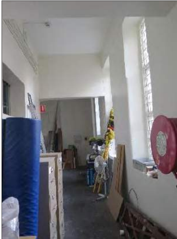
Figure 114: Room 308-309 in the CMP 2016 . This hallway has plastered walls with a dado line and a concrete ceiling.
