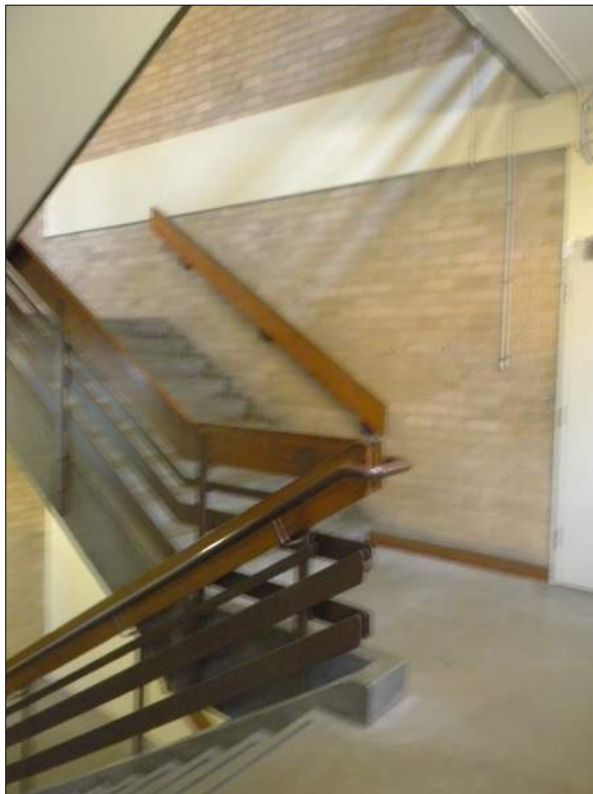
Figure 137: Typical stairwell within building 4, showing concrete stair and timber and metal balustrade.
