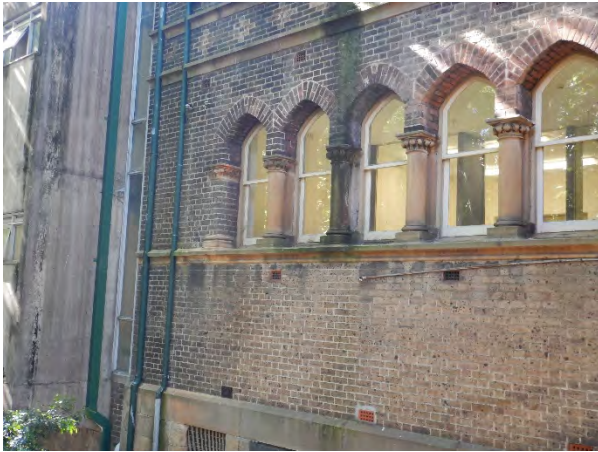
FIGURE 4.37 SOUTH FAÇADE OF BUILDING 2A, WHERE IT CONNECTS TO BUILDING 4 SHOWING SPALLING AND STAINING OF MASONRY FABRIC.
