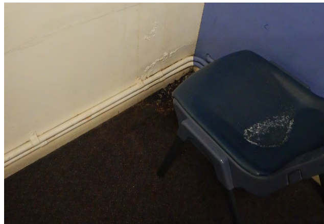
FIGURE 4.25 WATER INGRESS IN ROOM 172 HAS ALSO CAUSED DAMAGE TO WALL AND FLOOR FABRIC.
