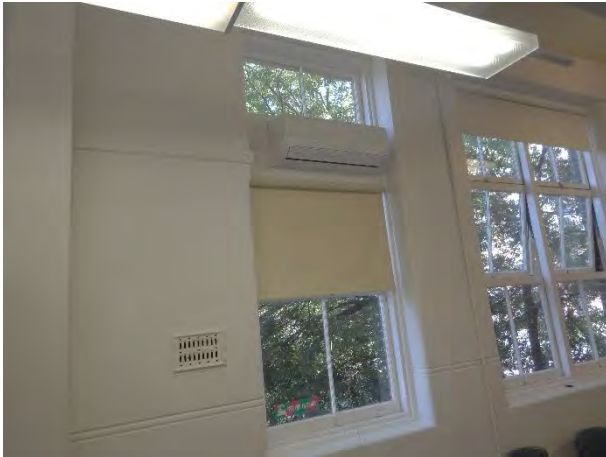
FIGURE 4.59 'WALL MOUNTED' AIR CONDITIONING UNIT ON GROUND FLOOR NORTHERN WINDOWS. PENETRATIONS HAVE BEEN MADE TO THE TIMBER FRAME TO CONNECT THE CONDUIT TO THE EXTERNAL RISER.
