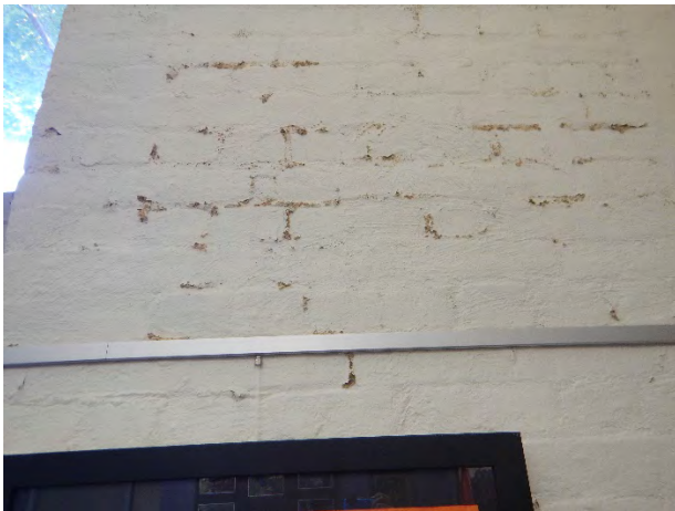
FIGURE 4.45 EFFLORESCENCE ON BRICK MASONRY WALL IN GROUND FLOOR RECEPTION, BUILDING 2A (ROOM G205).
