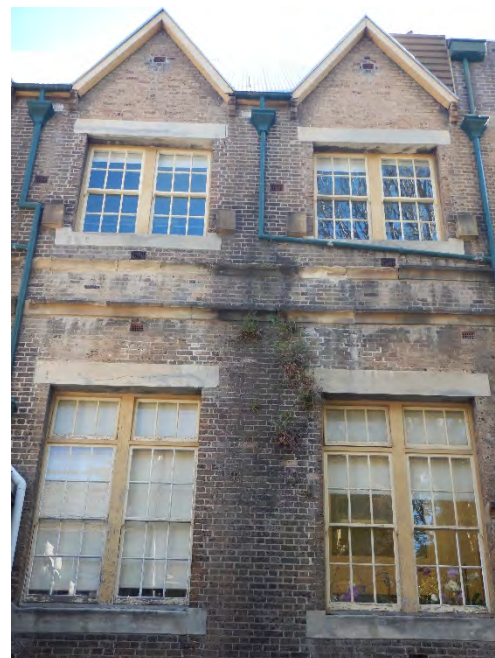
FIGURE 4.36 THE FABRIC OF THE NORTH ELEVATION OF BUILDING 2A TO THE WEST OF THE WALKWAY IS IN POOR CONDITION, WITH SEVERELY SPALLING SANDSTONE (INCLUDING STRING LINES) AND BRICKWORK. A RANGE OF SELF-SEEDING VEGETATION IS ALSO PRESENT.
