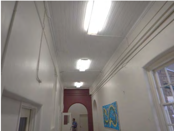
FIGURE 4.18 SURFACE MOUNTED CONDUITS ARE PRESENT ON CEILINGS AND WALLS WITHIN A MAJORITY OF SPACES IN BUILDING 1. THIS EXAMPLE SHOWS THE CORRIDOR ON THE GROUND FLOOR.
