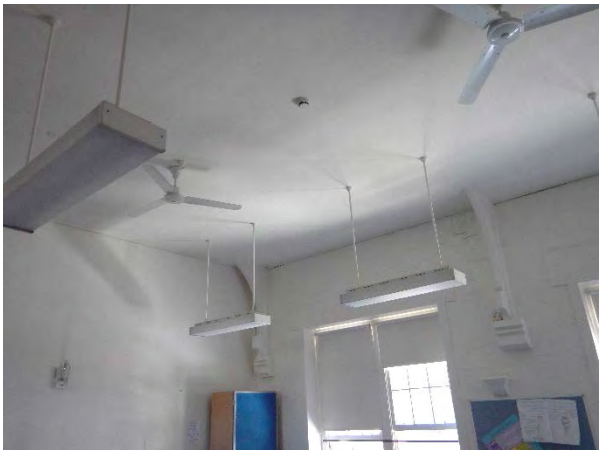
FIGURE 4.41 INFILL CEILINGS WITHIN CLASSROOM. NOTE CORBELS AND BASE OF TRUSS STRUCTURE, WHICH SUGGESTS THAT A FLOOR WAS INTRODUCED ABOVE.
