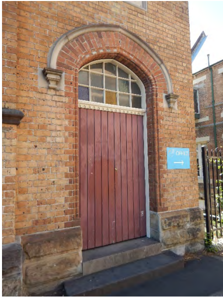
FIGURE 4.16 EXTERNAL PAINTED TIMBER SURFACES WILL REQUIRE REPAINTING IN THE MEDIUM TERM TO PROTECT TIMBER FABRIC. THIS EXAMPLE IS THE CHALMERS ST ENTRANCE DOOR.
