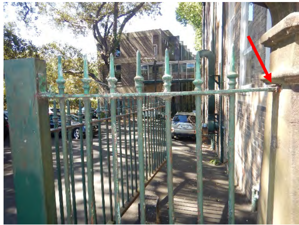
FIGURE 4.15 EARLY PALISADE FENCE ADJACENT TO BUILDING 1B REQUIRES RUST TREATMENT AND PAINTING MAINTENANCE. NOTE RUSTING WHERE SET INTO STONE PIER WILL ALSO AFFECT STONEMASONRY.
