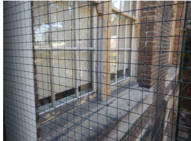
FIGURE 4.38 TIMBER FABRIC, INCLUDING WINDOW FRAMES AND SASHES, REQUIRE PROTECTION VIA PAINTING MAINTENANCE WORKS AS THE CURRENT FINISHES HAVE SEVERELY DETERIORATED. THIS EXAMPLE SHOWS FIRST FLOOR WINDOWS OF THE NORTH ELEVATION.
