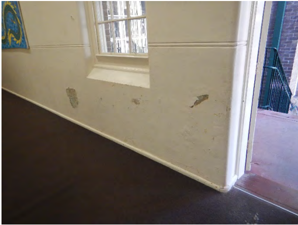
FIGURE 4.22 DRUMMY RENDER AND BLISTERING PAINT IN GROUND FLOOR CORRIDOR (SPACE 140).
