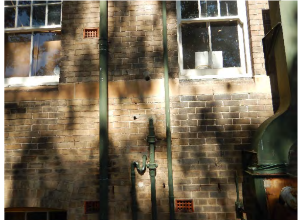
FIGURE 4.13 PENETRATIONS INTO THE MASONRY FABRIC FROM EXTERNALLY MOUNTED SERVICES, INCLUDING THOSE REMAINING WHERE SERVICES HAVE BEEN REMOVED.
