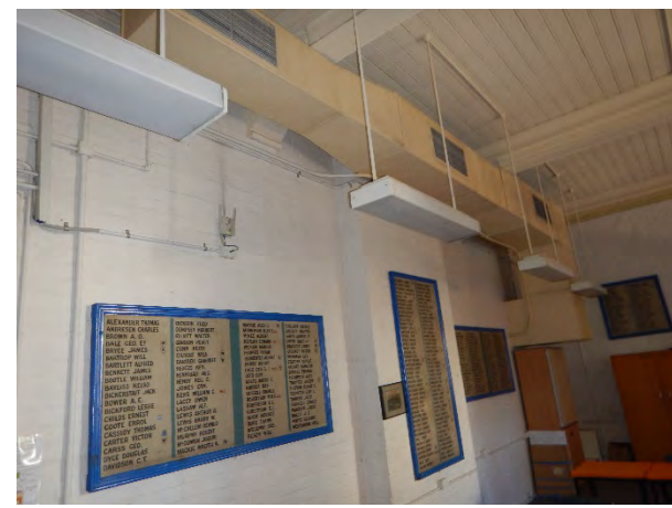
FIGURE 4.44 AIR CONDITIONING DUCT AND SUSPENDED SERVICES IN CLASSROOM (ROOM G212).
