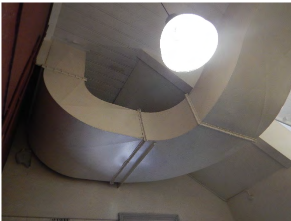
FIGURE 4.20 AIR CONDITIONING DUCTWORK WITHIN SOUTHERN STAIRWELL (SPACE 130).
