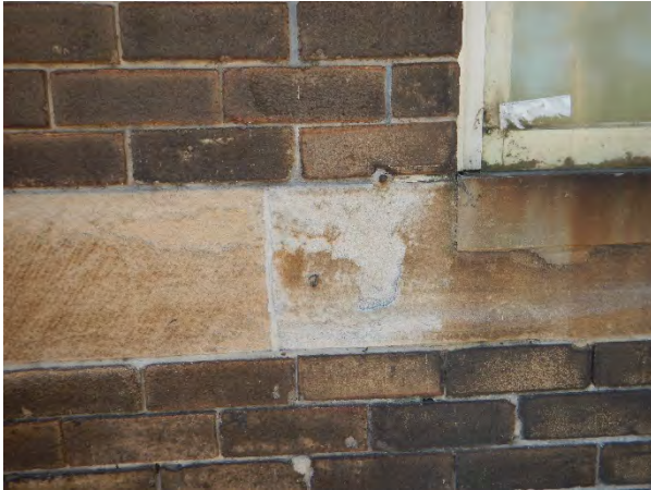
FIGURE 4.12 EXAMPLE OF SPALLING SANDSTONE SILL ON THE CLEVELAND ST ELEVATION OF THE 1909 BUILDING.
