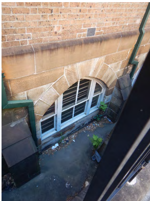
FIGURE 4.35 VIEW OF LOWER GROUND SANDSTONE FABRIC FACING CHALMERS STREET, SHOWING STAINING.
