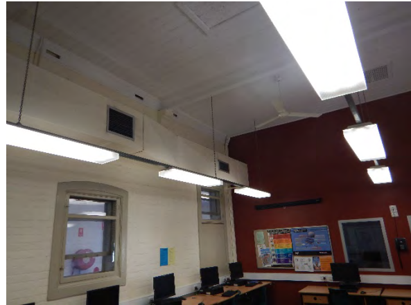
FIGURE 4.19 AIR CONDITIONING DUCT, WHICH IS TYPICAL IN ROOMS ALIGNED ADJACENT TO CLEVELAND STREET. NOTE ALSO THE CEILING FAN, WHICH IS TYPICAL THROUGHOUT BUILDING 1.
