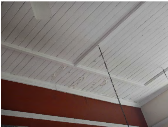
FIGURE 4.24 EXAMPLE OF PEELING AND FLAKING PAINT ON TIMBER BOARDED CEILINGS IN BUILDING 1.
