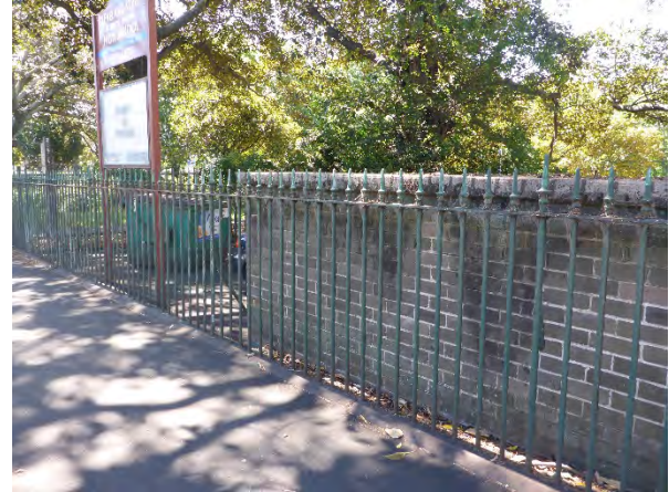
FIGURE 4.3 EARLY PALISADE FENCE SET INTO STONE BASE EXTENDING ALONG THE CLEVELAND STREET BOUNDARY.
