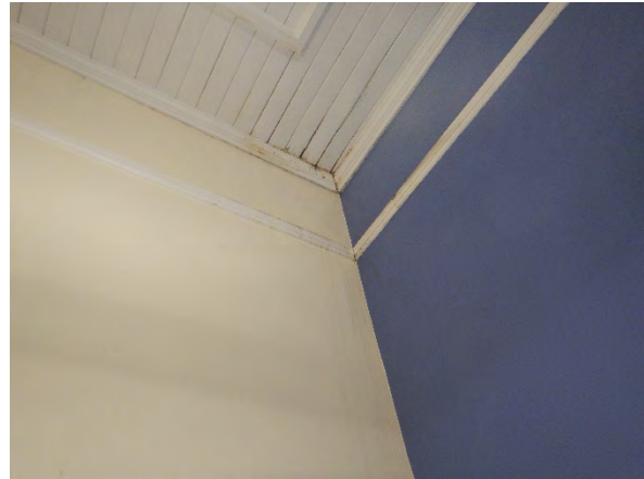
FIGURE 4.23 WATER DAMAGE TO CEILING AND STAINING TO WALL IN FIRST FLOOR ROOM 172.
