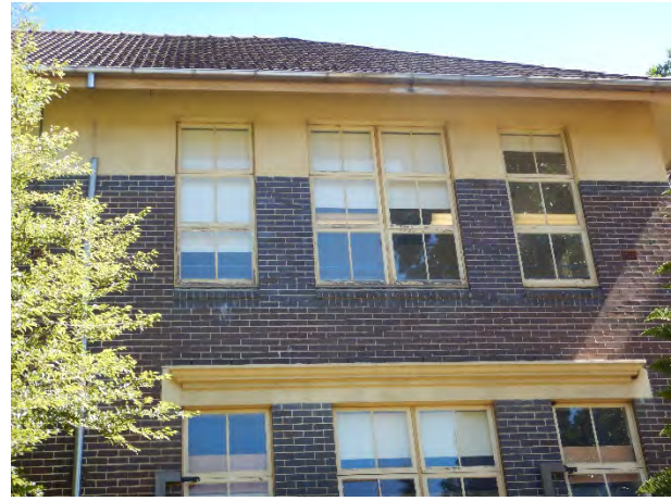
FIGURE 4.52 EXTERNAL PAINTED FINISHES ARE DETERIORATING CONSIDERABLY, INCLUDING WINDOW FRAMES, EAVES AND FASCIAS.
