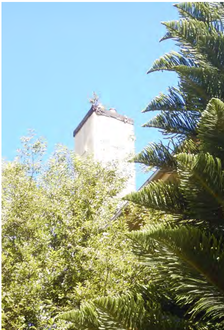
FIGURE 4.53 SELF-SEEDING VEGETATION ON NORTHERN CHIMNEY.
