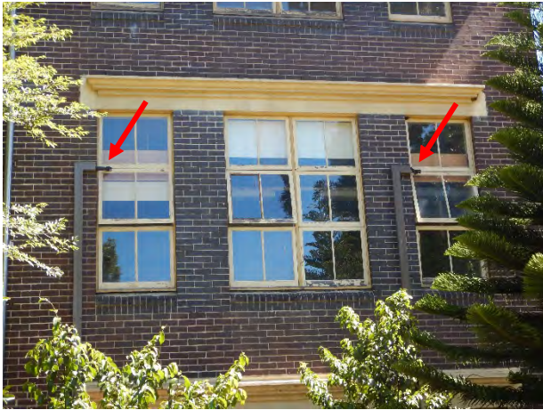
FIGURE 4.51 PARTIAL VIEW OF NORTH ELEVATION SHOWING EXTERNALLY MOUNTED AIR CONDITIONING RISERS, WITH CONDUITS PENETRATING TIMBER WINDOW FRAMES (SHOWN BY RED ARROWS).
