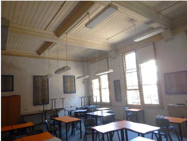
FIGURE 4.39 COFFERED TIMBER CEILINGS WITHIN CLASSROOM (ROOM G212).
