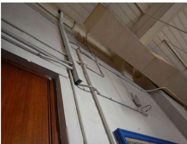
FIGURE 4.43 AN ARRAY OF SURFACE MOUNTED SERVICES HAVE BEEN ATTACHED TO BOTH WALLS AND CEILINGS.
