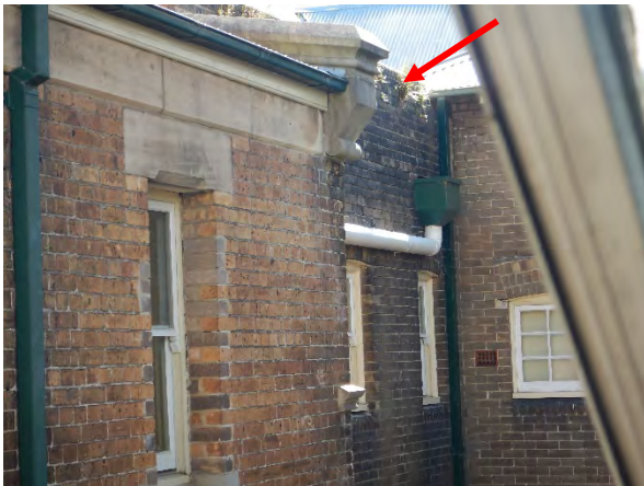
FIGURE 4.14 VEGETATION GROWING ON THE UPPER LEVEL OF THE BUILDING (SHOWN BY RED ARROW).
