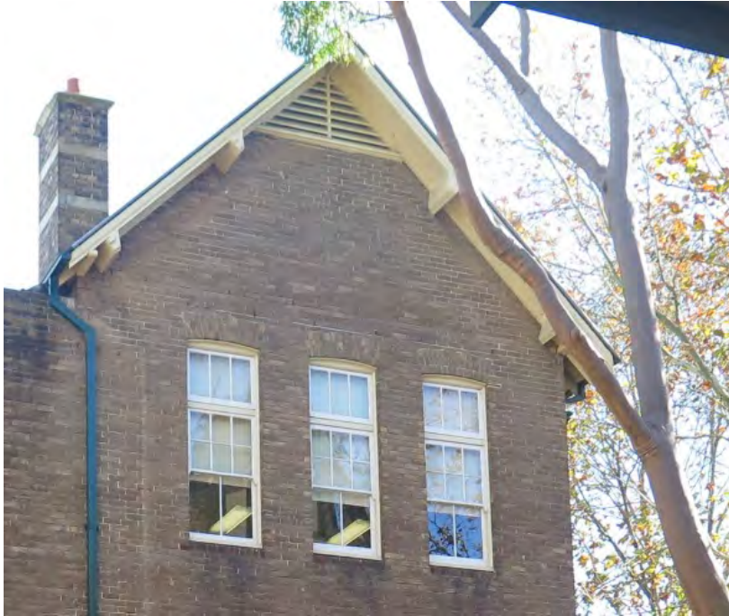
FIGURE 4.10 VIEW SHOWING THE GABLE END ON THE NORTH ELEVATION OF BUILDING 1B (1909) WHICH FEATURES FINE TIMBER WORK WITH A VENT INTO THE ROOF SPACE AS SEEN FROM THE SOUTH EAST COURTYARD. SOURCE: OCP ARCHITECTS, 2016.
