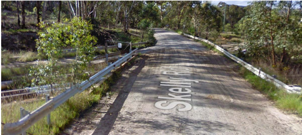
Figure 3.2 Pipeline passing within existing culvert under Skelly Road
