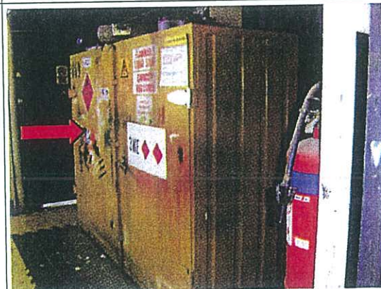
Photo 10. Yellow lead containing paint on paint storage container, Paint workshop, Level 3.
