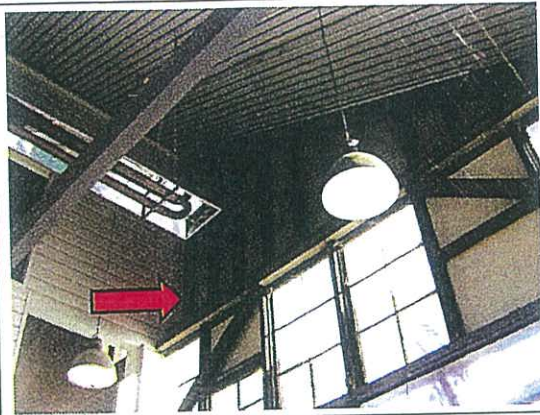
Photo 1. Upper wall panels, Level 3, Restaurant (Wharf) – Asbestos fibre-cement sheeting
