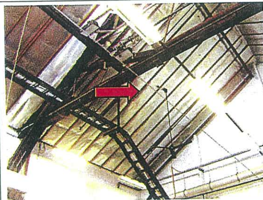
Photo 8. SMF sarking insulation to ceilings throughout building
