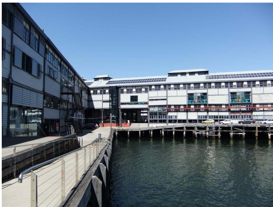
Photo 2: View looking south-west with shore sheds to the left of photo and east elevation of Wharf 4/5 to the right.
