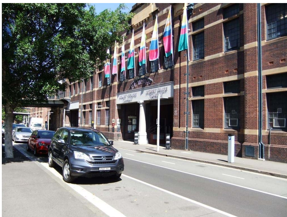
Photo 1: Shore sheds along Hickson Road showing entry to STC and Wharf 4/5
