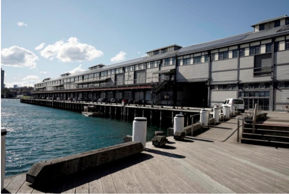
Photo 4: West elevation of Wharf 4/5
