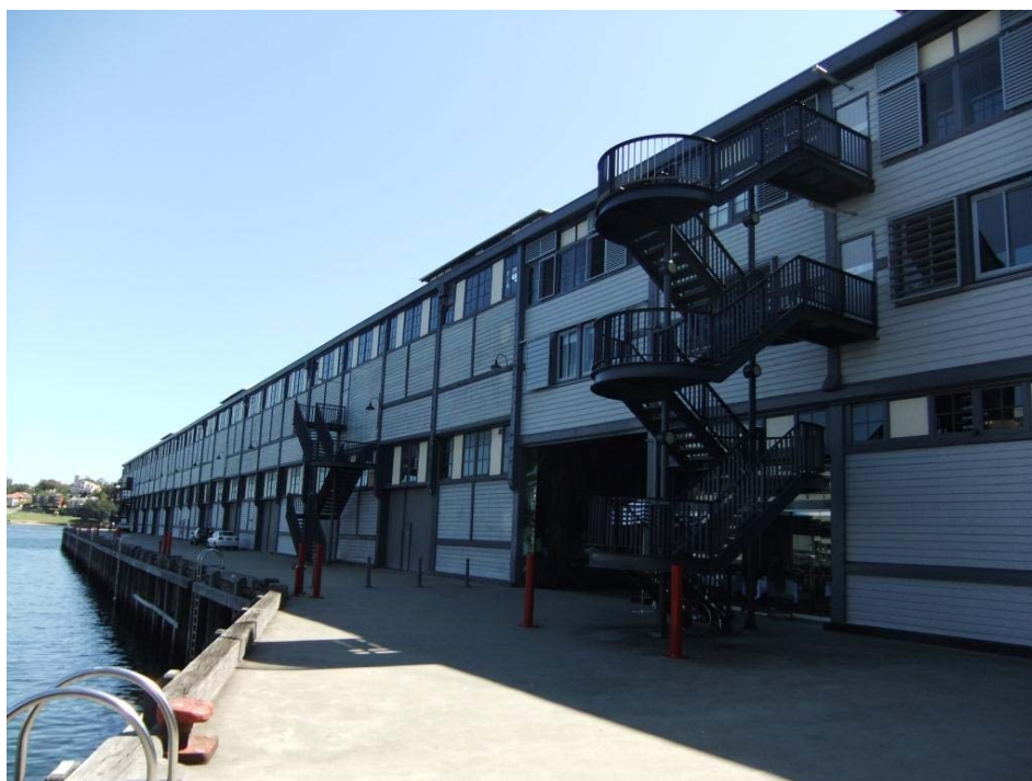
Photo 7: Pier 2/3 to the east
