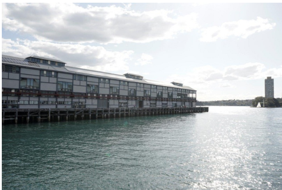
Photo 3: East elevation of Wharf 4/5
