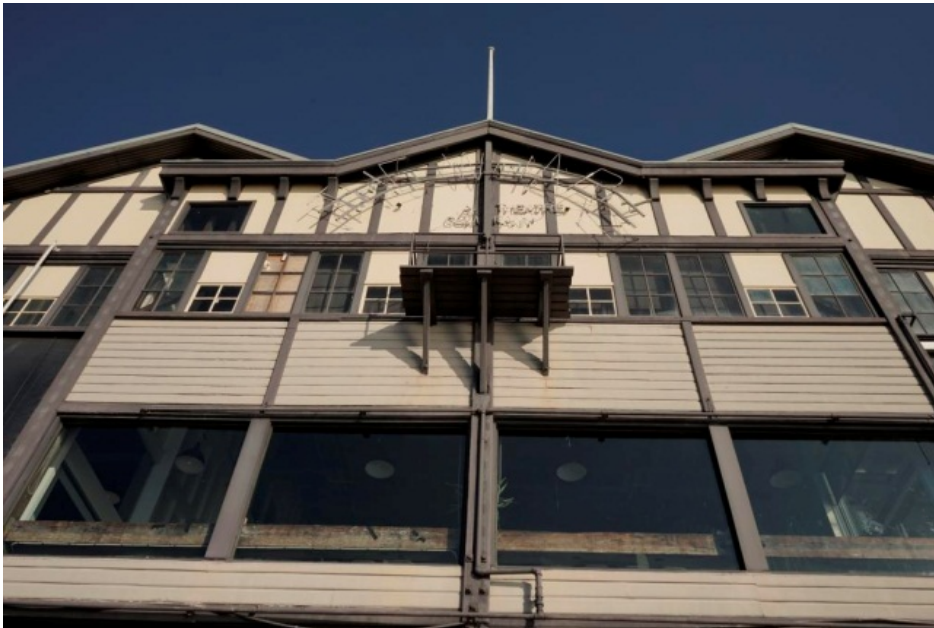
Photo 5: North elevation of Wharf 4/5
