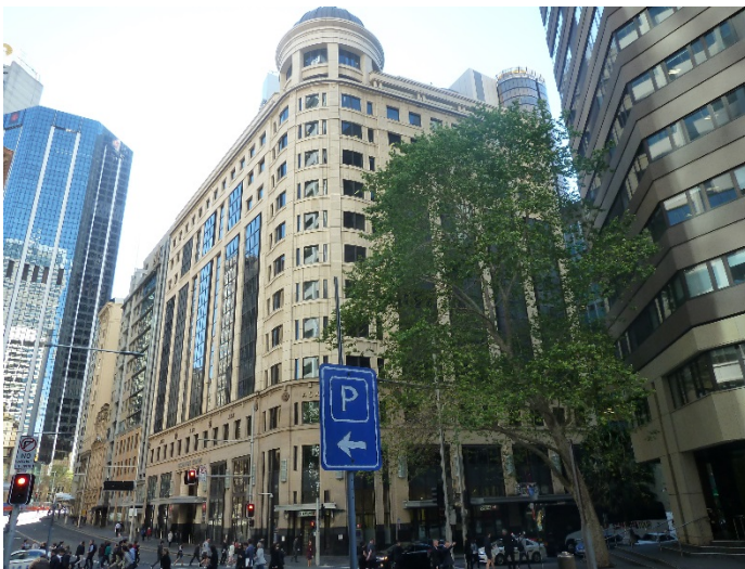
Figure 37 – Australian Stock Exchange building Source: JBA
