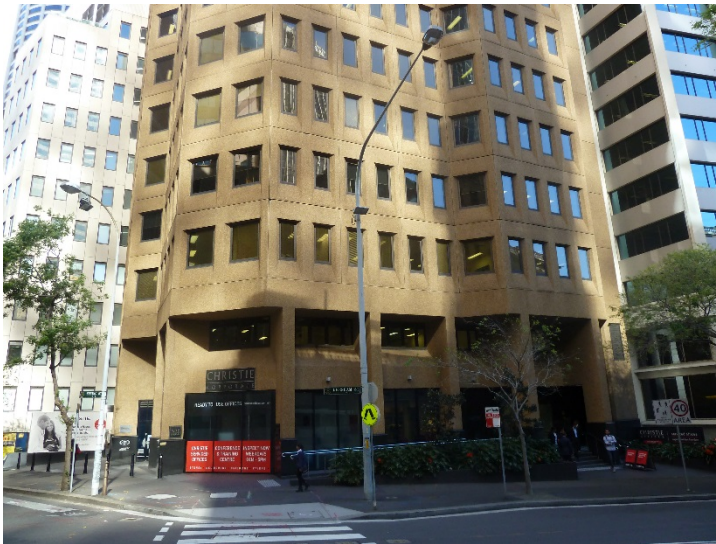
Figure 36 – Christie Conference Centre building Source: JBA
