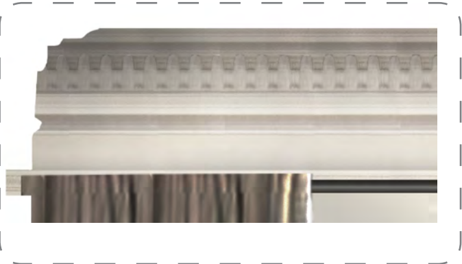
Detail of proposed painted cornice Existing cornice painted varying shades of neutral tones and gloss levels to highlight existing heritage detailing
