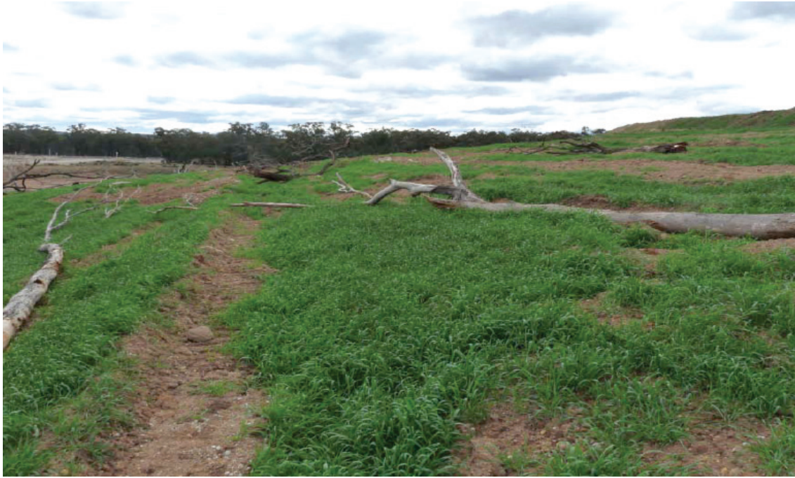
Plate 5-9 Tarrawonga Coal Mine - Northern Emplacement Following Reshaping, Fauna Habitat Placement and Cover Crop Establishment (2013)
