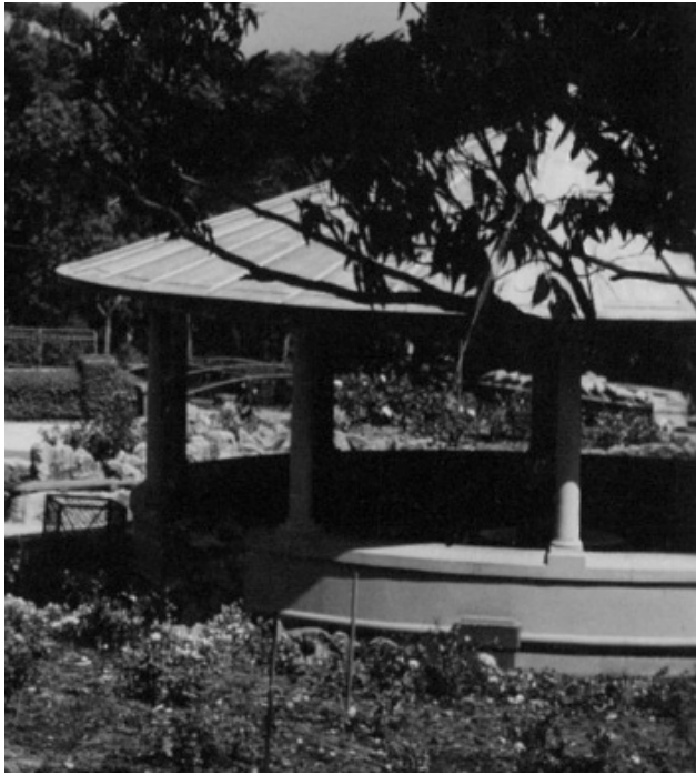
Historic image of shelter showing roof cladding detail and the wall prior to its infilling. The wall has an angled top and there is a block or column base under each column.
