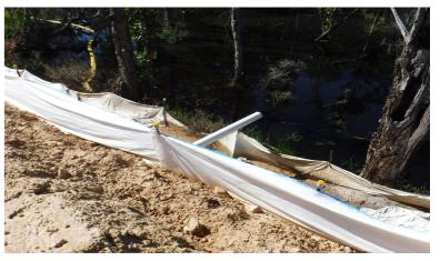
**Geofabric Double Apron Example** Stabilised Aggregate to be used to ground the toe of the Geofabric Apron.
