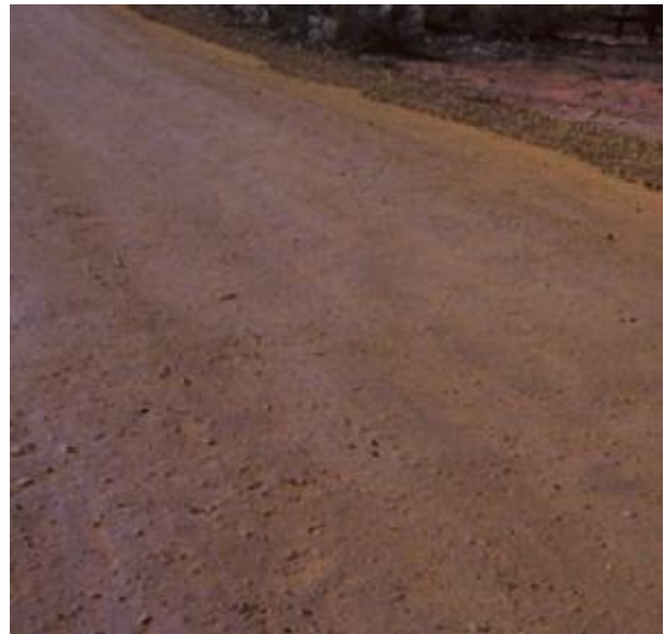
Picture 6 – After Application of Polymer Spray
