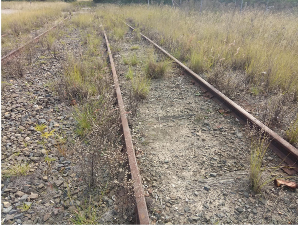
Photo (13): Existing train tracks in poor condition
