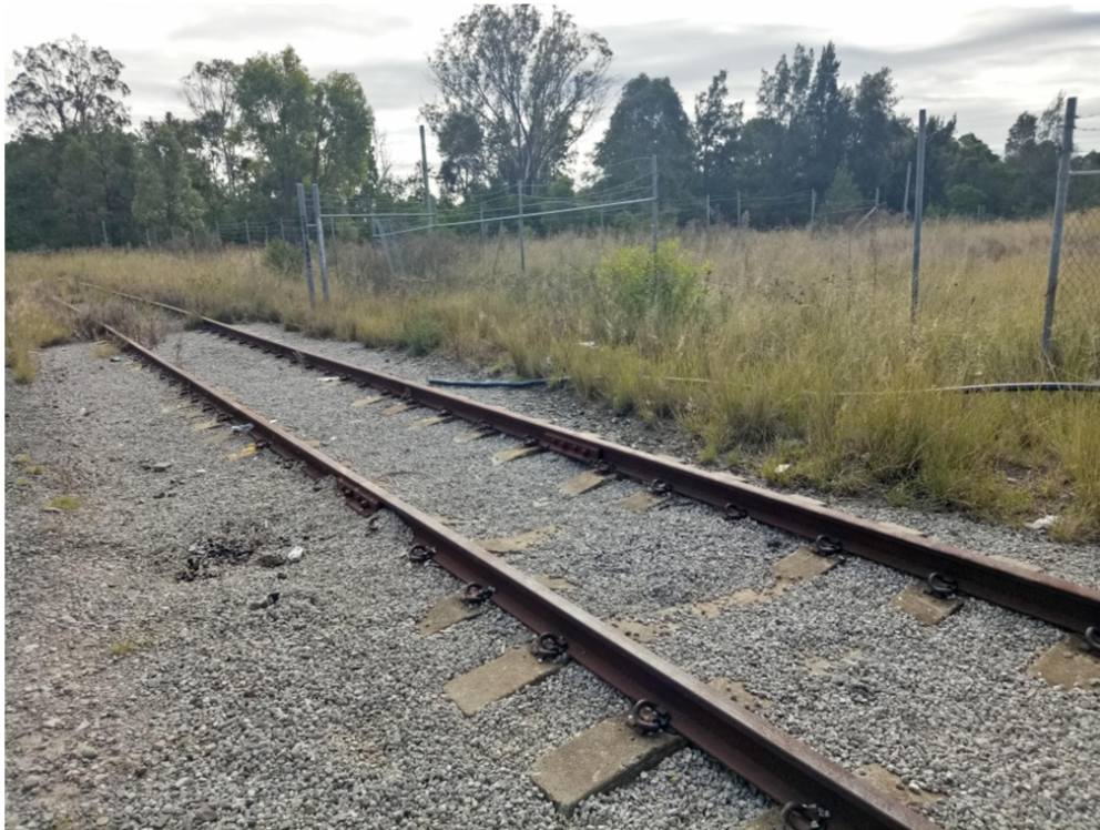
Photo (12): Existing train tracks in poor condition and existing damages in boundary fence
