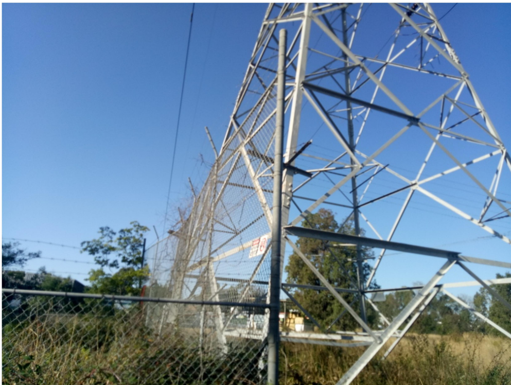
Photo (40): Existing lattice tower with poor condition fence
