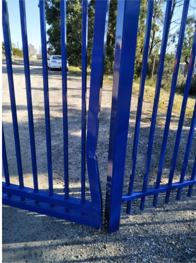
Photo (33): Existing damage in the entry gate from Forrester Road
