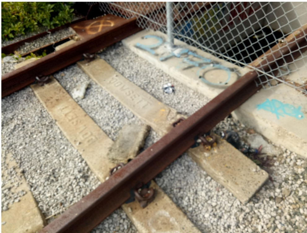
Photo (10): Existing train tracks in poor condition
