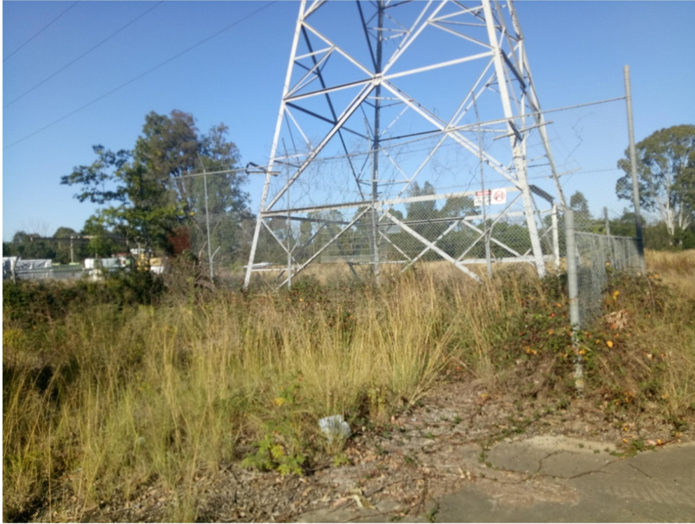
Photo (41): Existing lattice tower with poor condition fence
