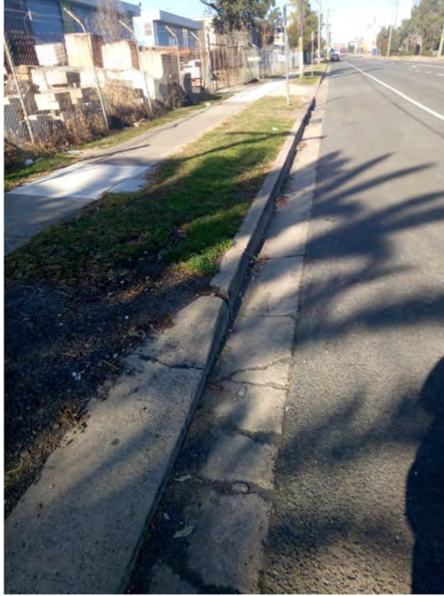
Photo (91): Existing damage in the kerb & gutter along Forrester road (site opposite side)
