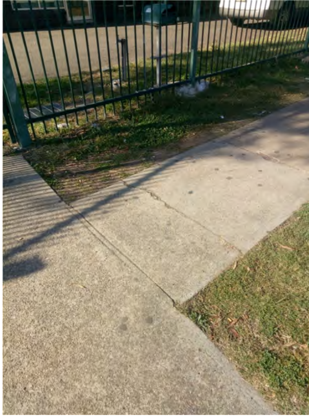
Photo (93): Existing damage in the footpath along Forrester road (site opposite side)
