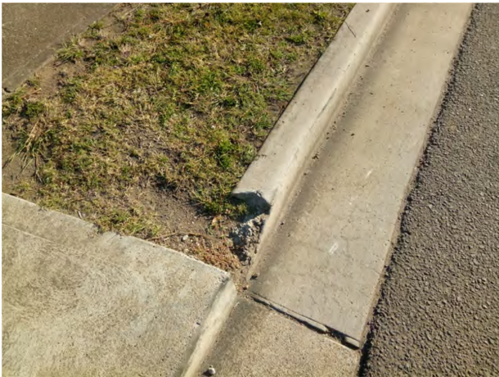
Photo (58): Existing cracks in St Marys manufacturing facilities entry kerb
