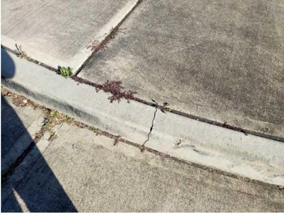
Photo (39): Existing cracks in the roundabout
