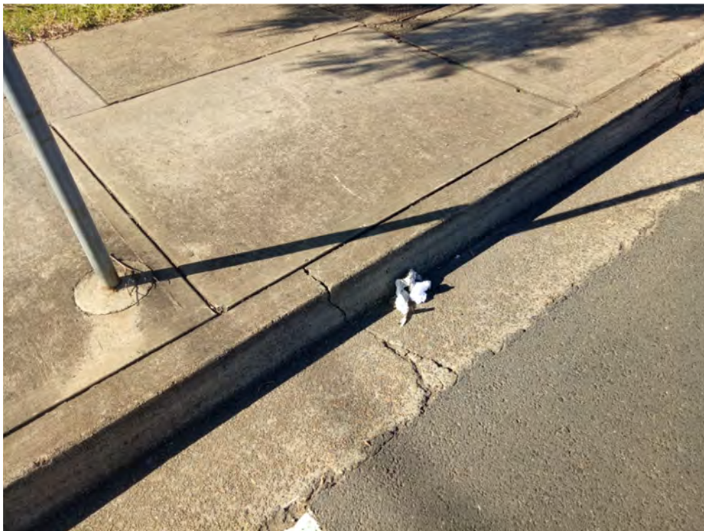
Photo (24): Existing cracks in the kerb & gutter in front of the site entry
