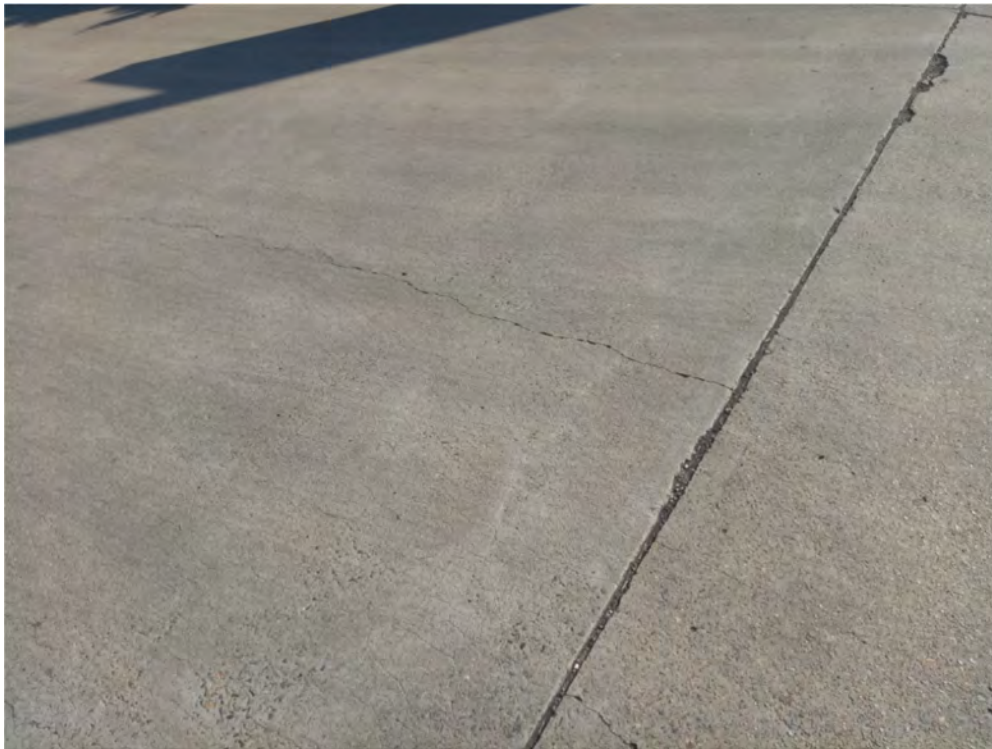
Photo (67): Existing damage/cracks at St Marys manufacturing facilities trucks entry
