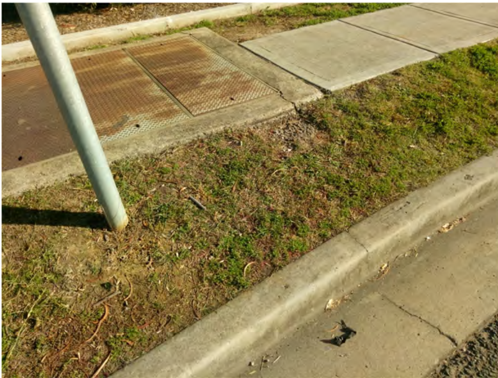
Photo (50): Existing damage/cracks in the kerb & gutter and footpath along Forrester road (site same side)
