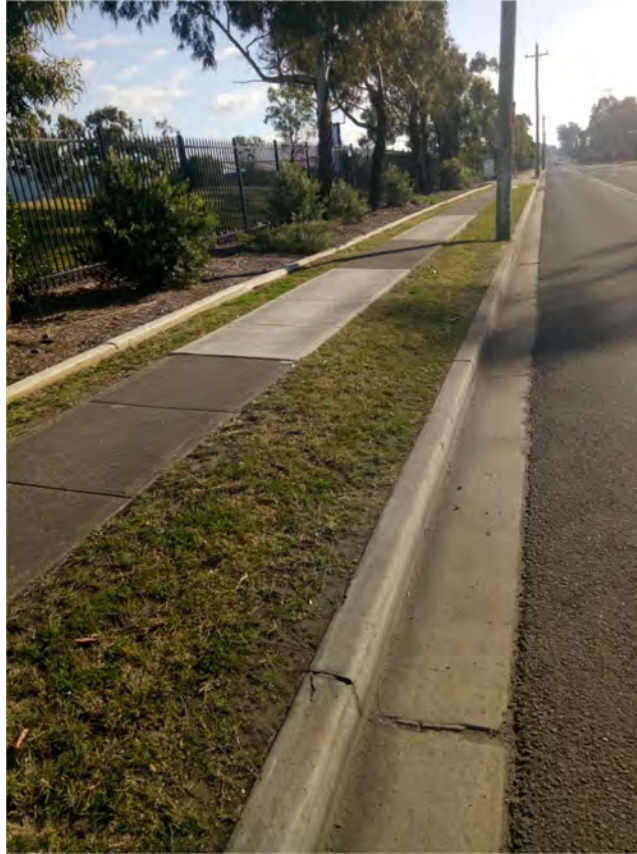
Photo (59): Existing cracks in the kerb & gutter along Forrester road (site same side)
