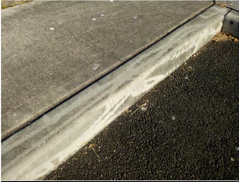
Photo (9): Existing cracks along the kerb adjacent to the site
