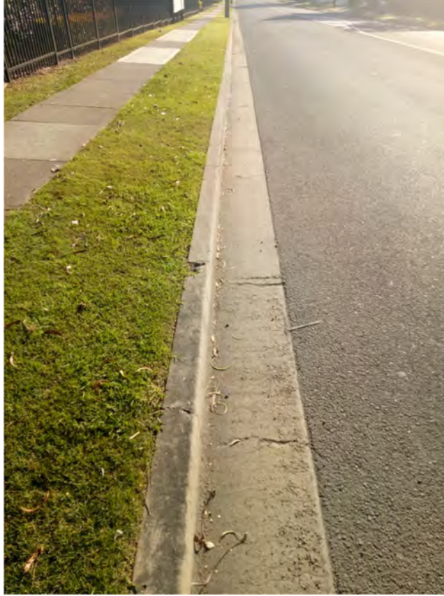
Photo (77): Existing damage in the kerb & gutter along Forrester road (site same side)
