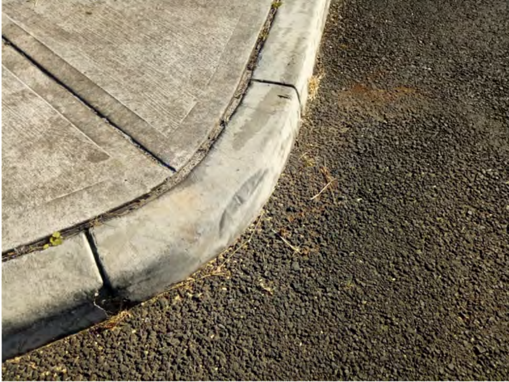
Photo (11): Existing damage in the kerb adjacent to the site
