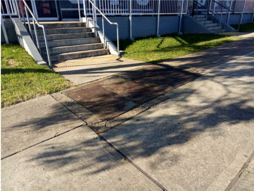
Photo (23): Existing cracks in the kerb & footpath in front of the site entry
