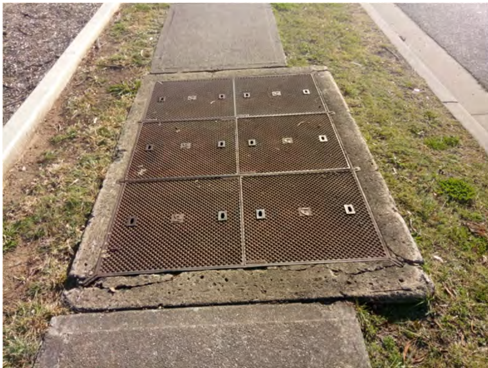
Photo (61): Existing cracks in the pit along Forrester road (site same side)
