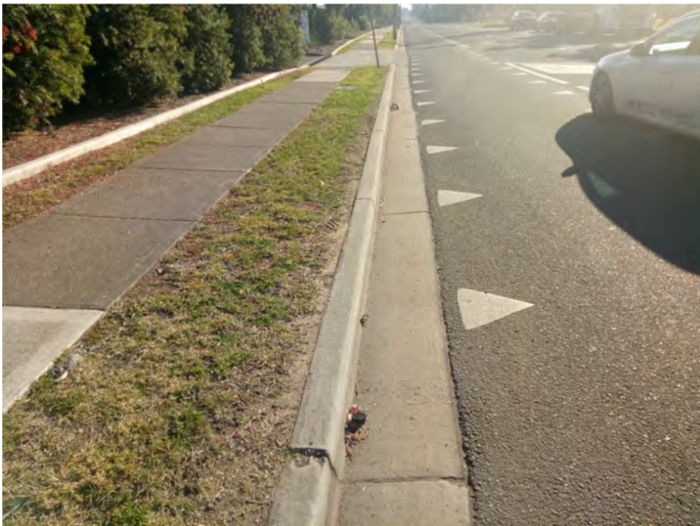
Photo (52): Existing damage/cracks in the kerb & gutter along Forrester road (site same side)
