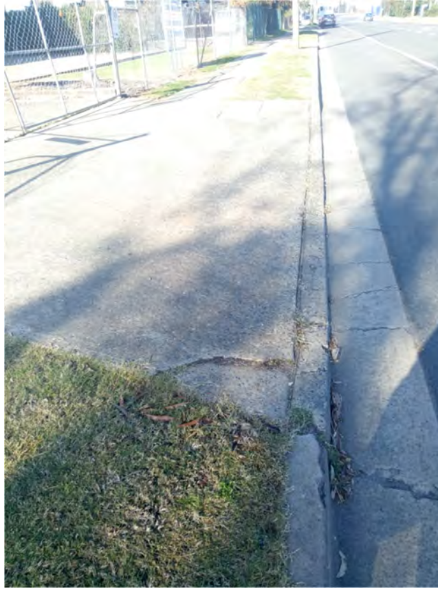
Photo (92): Existing damage in the kerb & gutter along Forrester road (site opposite side)
