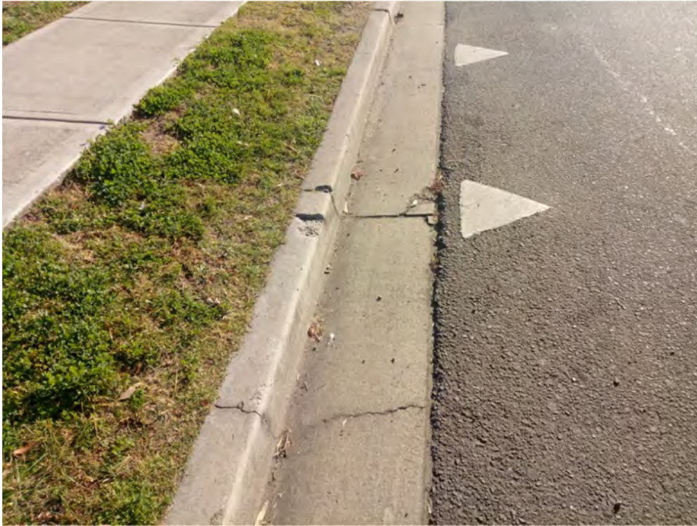
Photo (51): Existing damage/cracks in the kerb & gutter along Forrester road (site same side)
