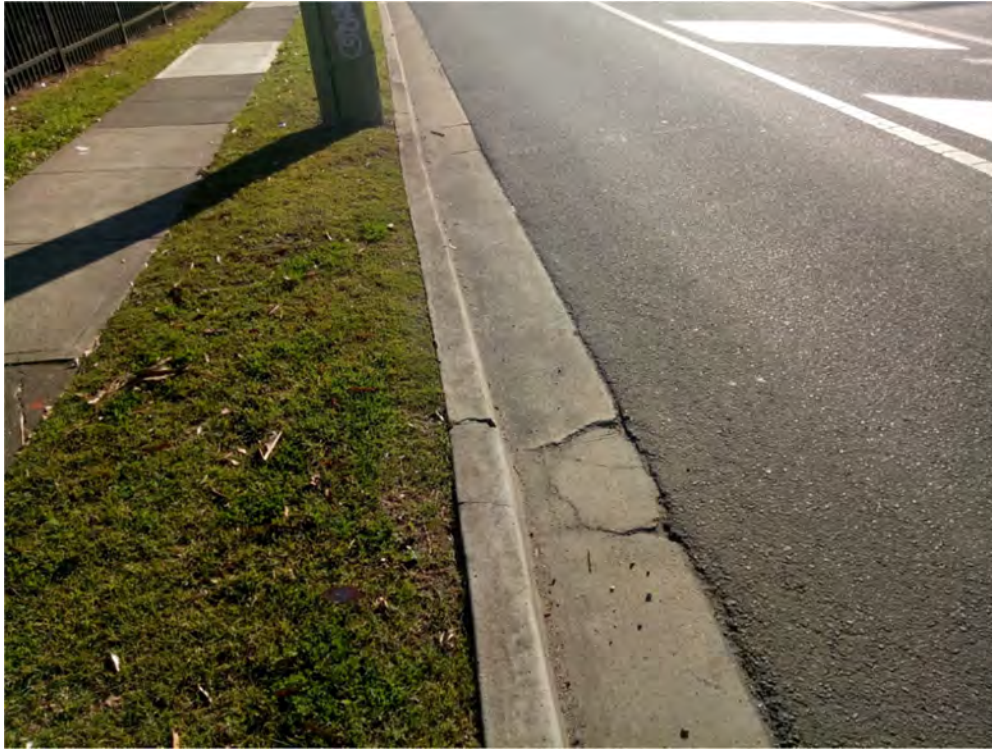
Photo (74): Existing damage/cracks in the kerb & gutter along Forrester road (site same side)
