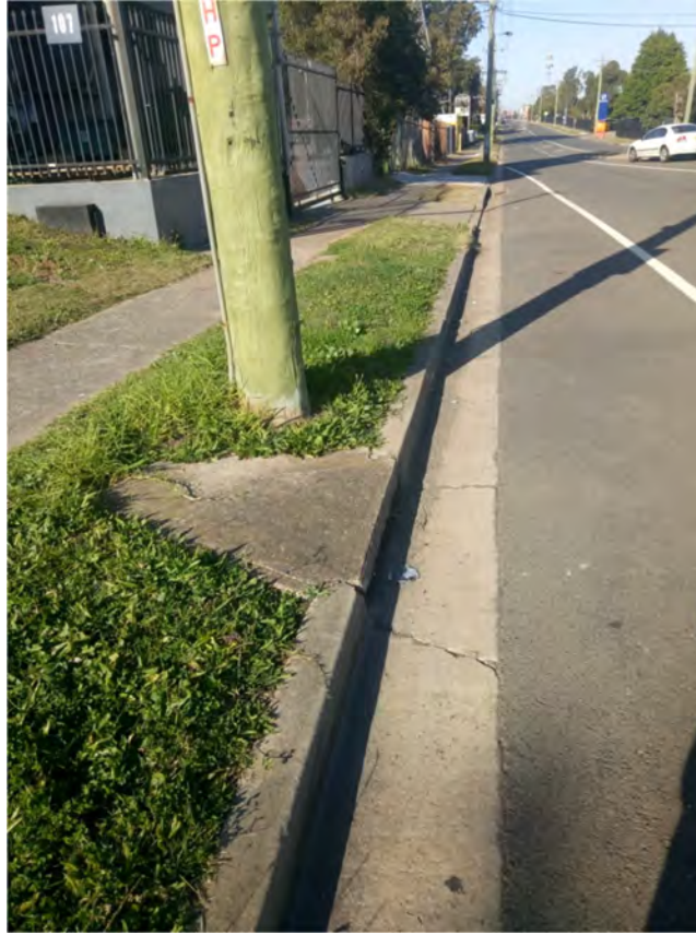
Photo (86): Existing damage in the kerb & gutter along Forrester road (site opposite side)
