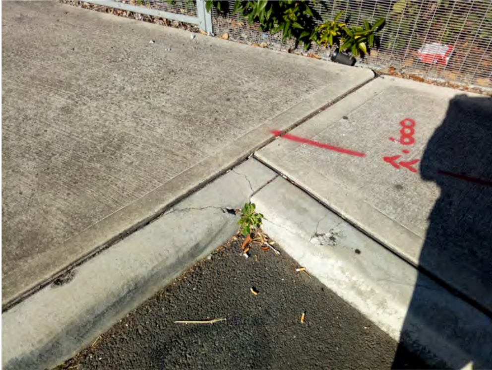
Photo (33): Existing cracks in the kerb at the roundabout area
