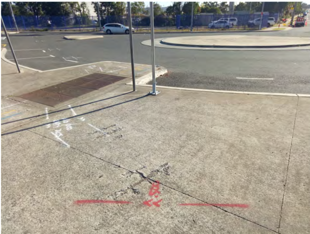
Photo (28): Existing damage in the footpath at the roundabout area
