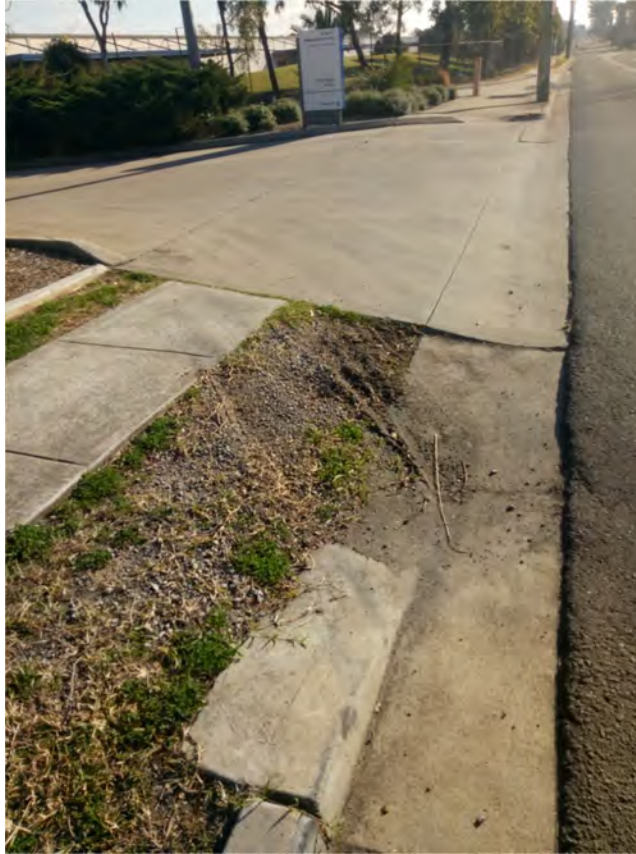
Photo (65): Existing damage in the kerb & gutter along Forrester road (site same side)
