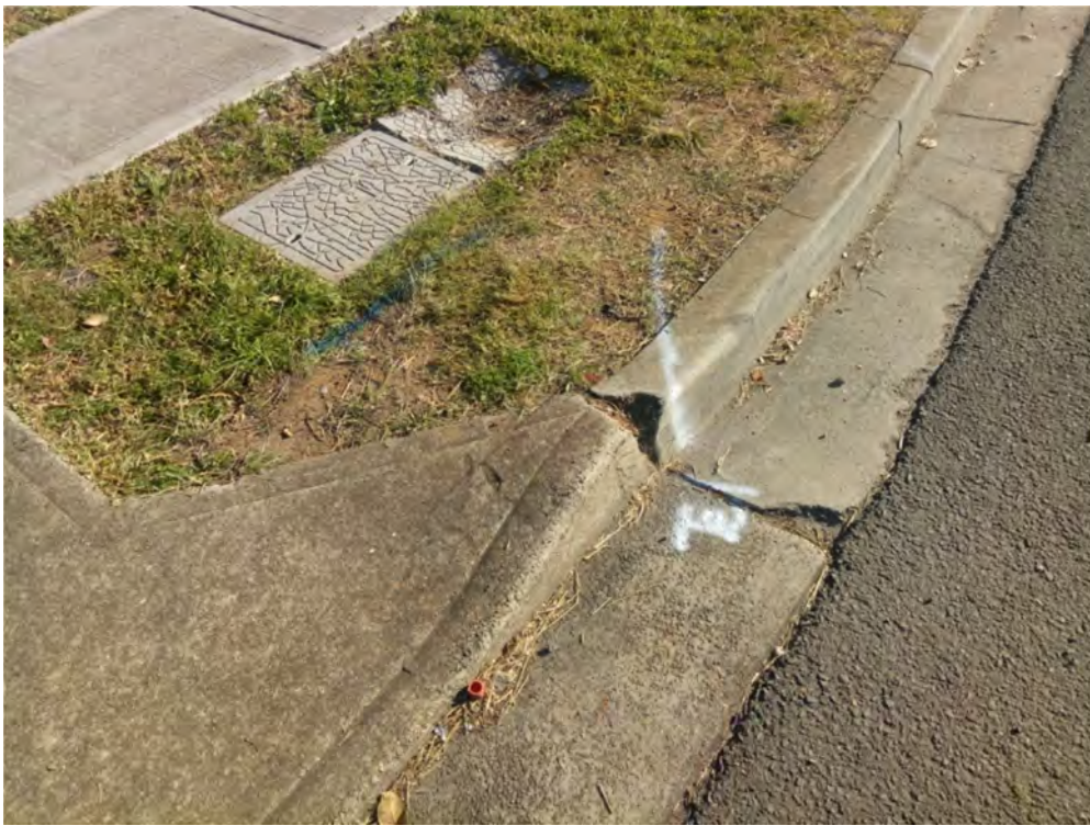
Photo (48): Existing damage in the kerb and pit cover at the driveway entry next to the site
