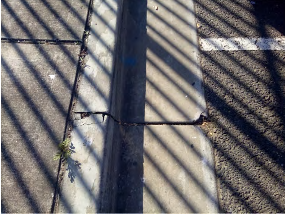
Photo (13): Existing damage in the kerb adjacent to the site
