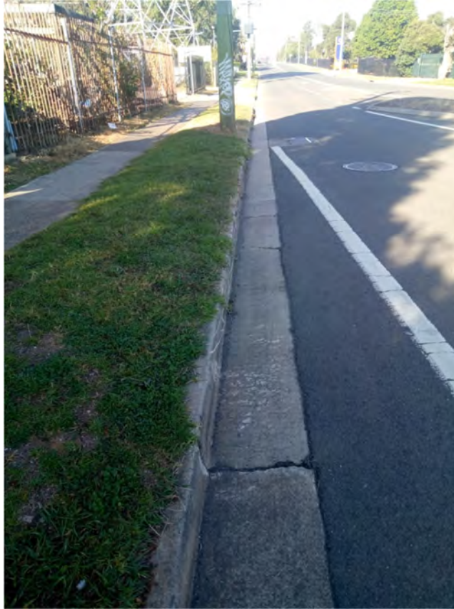
Photo (88): Existing damage in the kerb & gutter along Forrester road (site opposite side)
