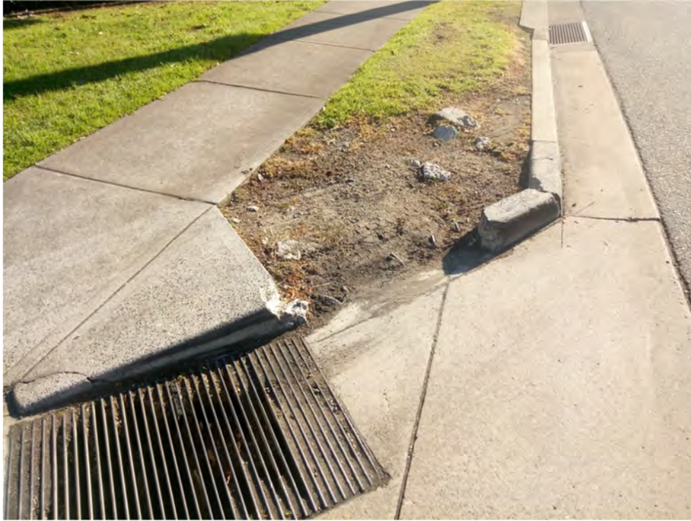
Photo (82): Existing damage in the kerb at Stockland entry along Forrester road (site same side)
