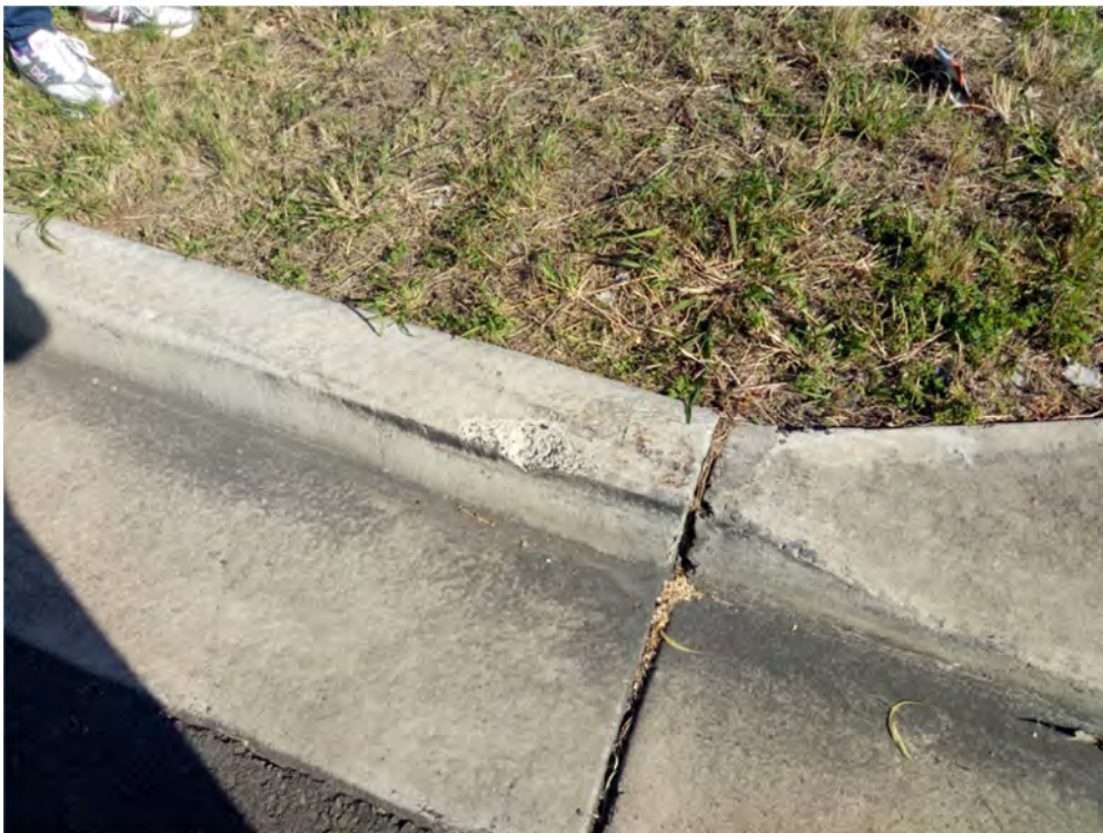
Photo (42): Existing damage in the kerb at the site entry
