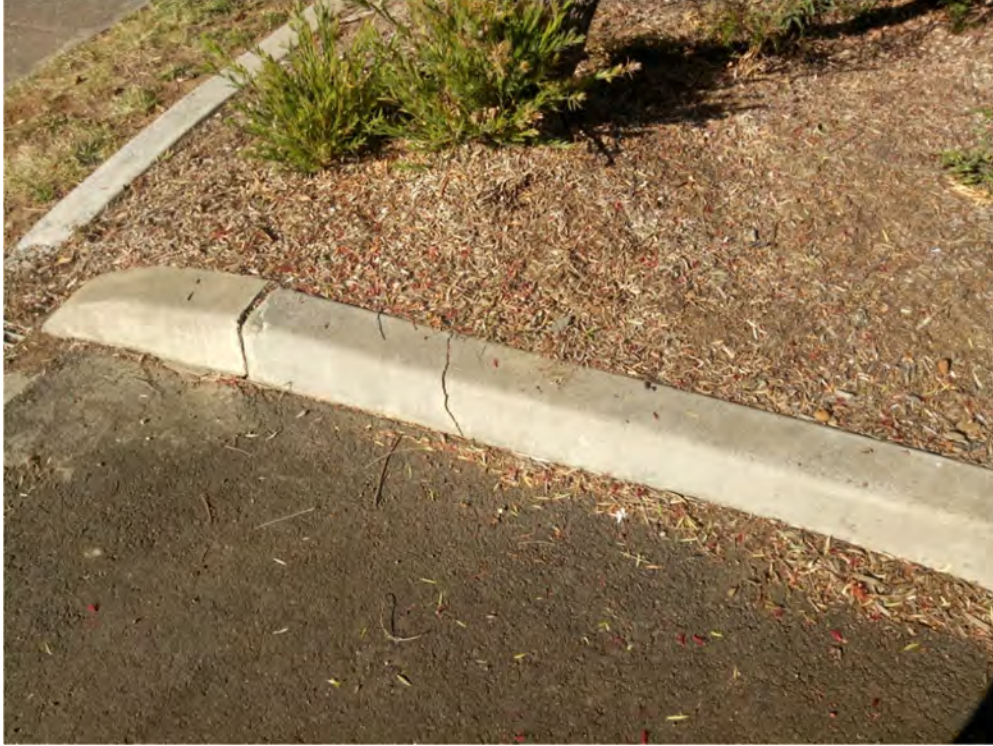
Photo (57): Existing cracks in St Marys manufacturing facilities entry
