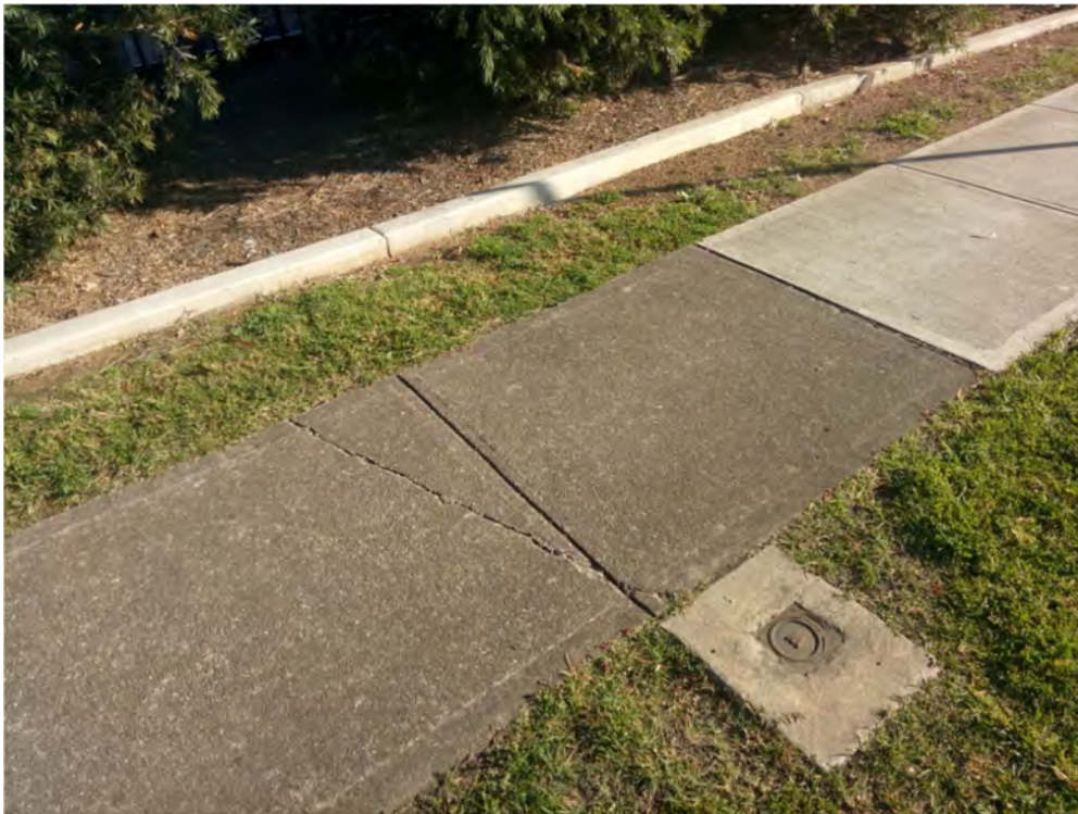
Photo (54): Existing cracks in the footpath along Forrester road (site same side)
