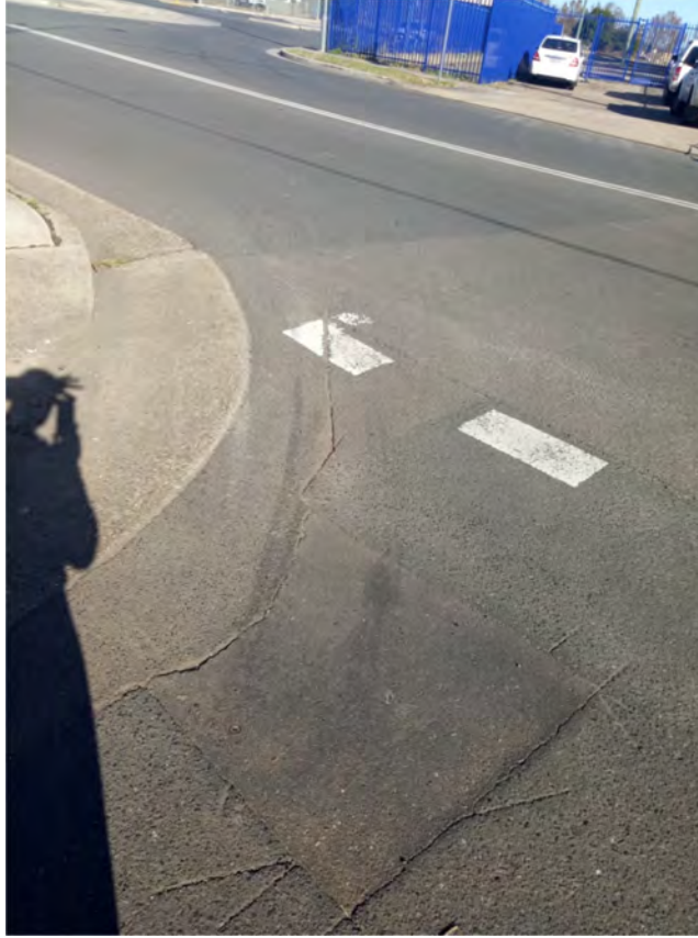
Photo (19): Existing damage/cracks in the road in front of the site entry
