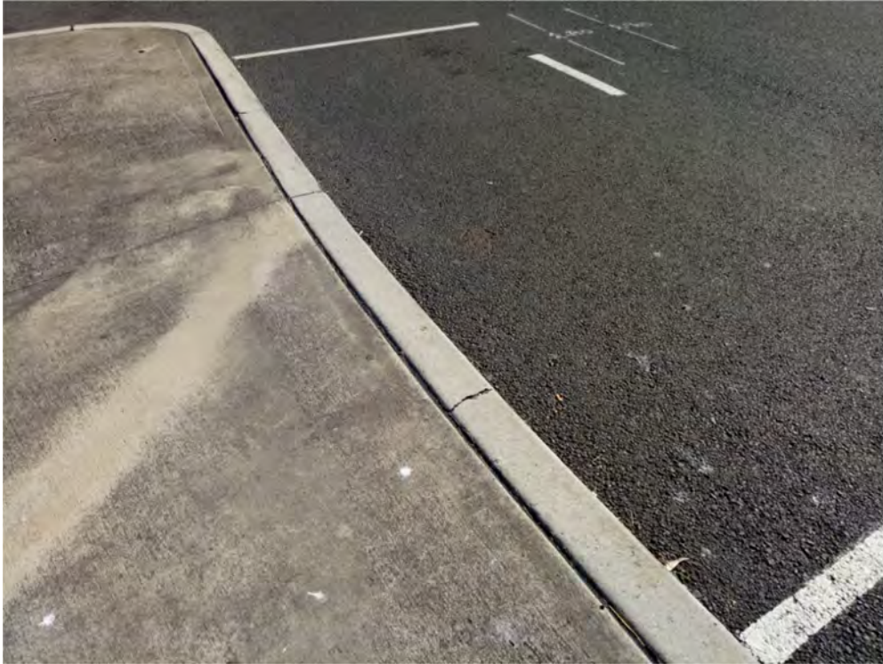
Photo (31): Existing cracks in the kerb at the roundabout area
