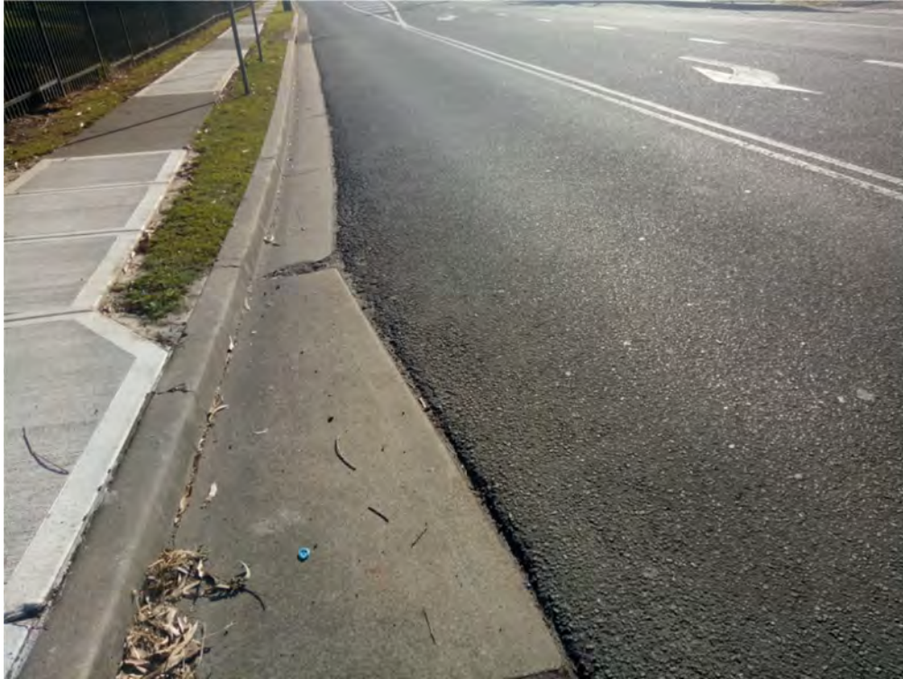
Photo (72): Existing damage/cracks in the kerb & gutter along Forrester road (site same side)
