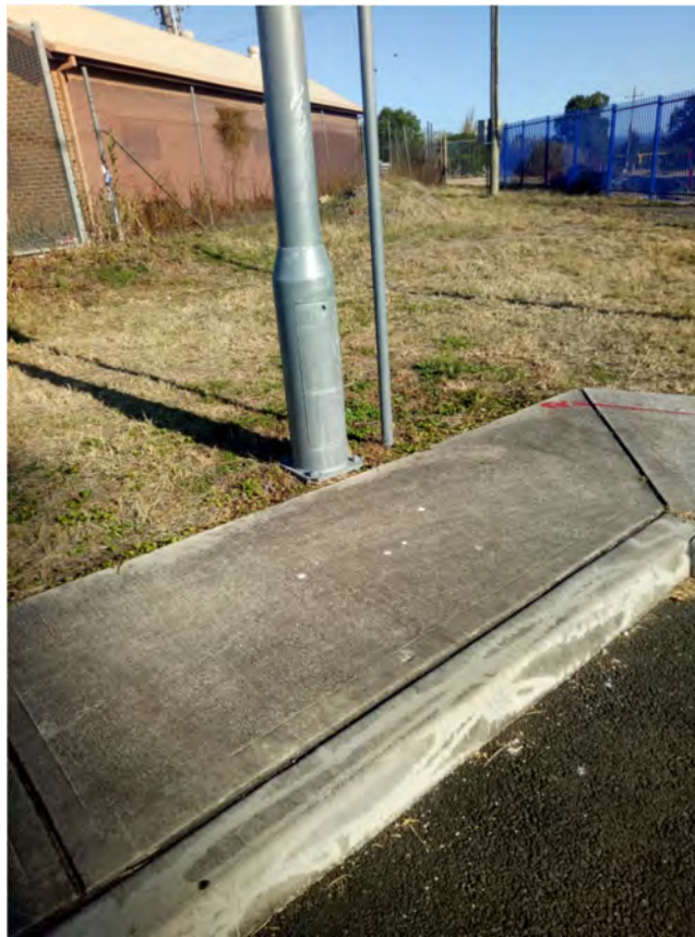
Photo (8): Existing cracks along the kerb adjacent to the site
