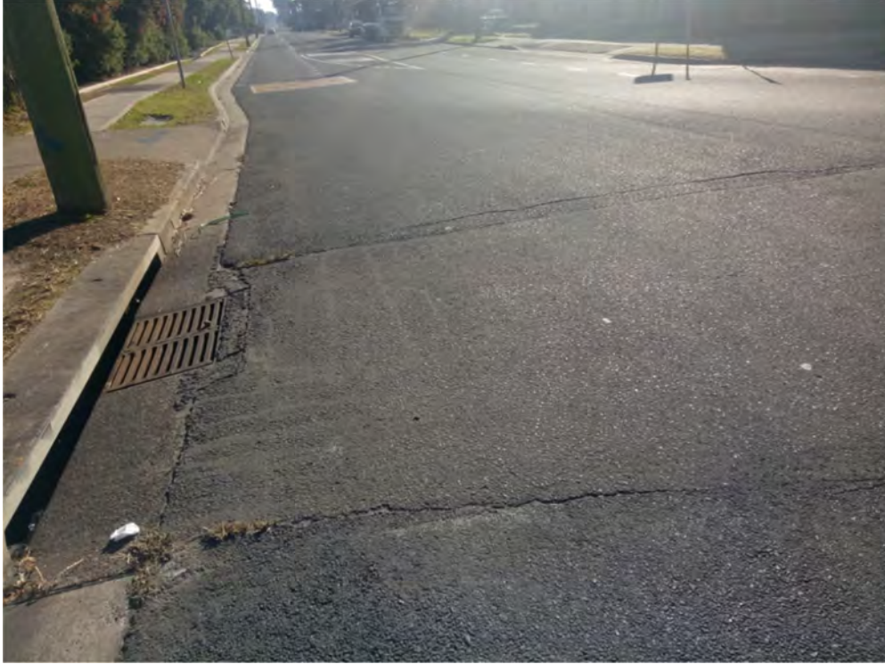
Photo (45): Existing damage/cracks in the road in front of the site entry
