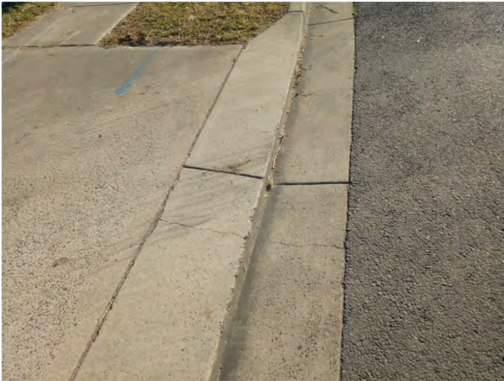
Photo (44): Existing crack in the kerb & gutter at the site entry
