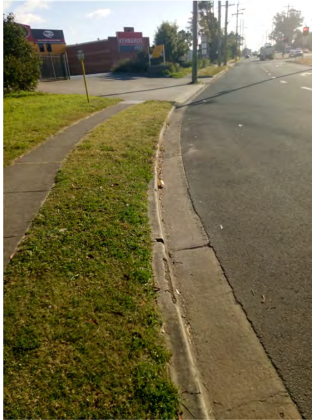
Photo (84): Existing damage in the kerb & gutter along Forrester road (site same side)
