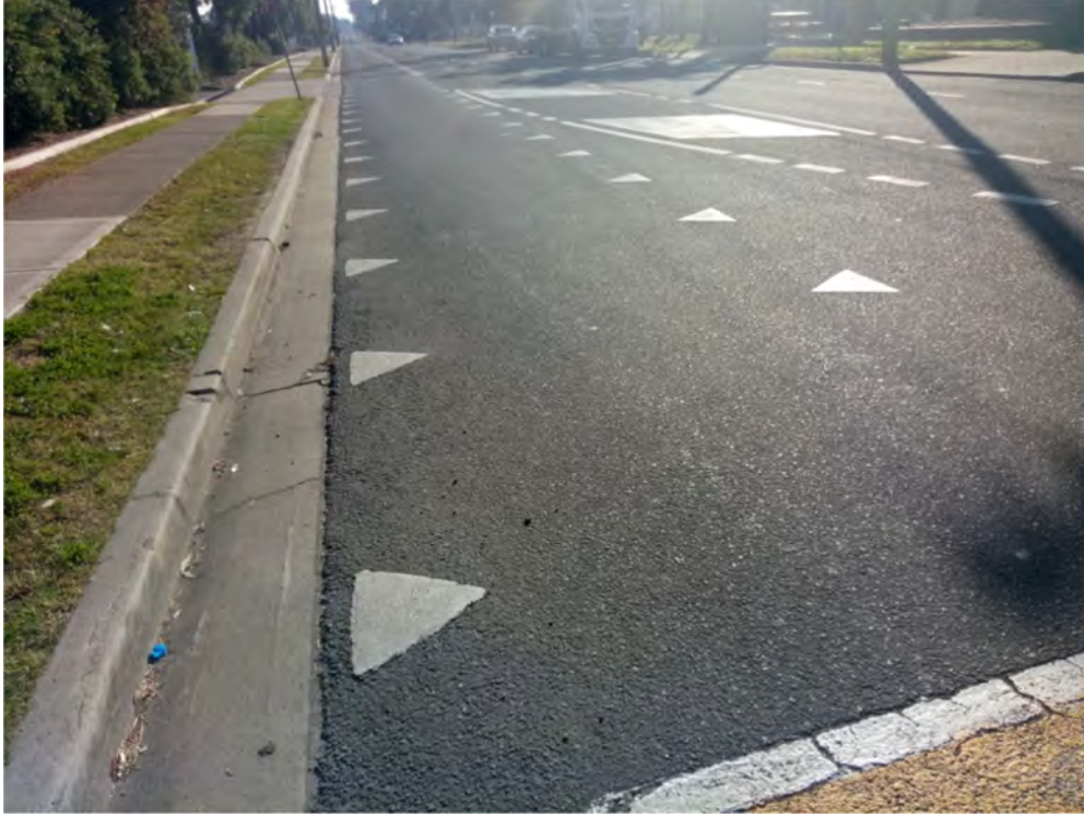
Photo (49): Existing damage/cracks in the kerb & gutter along Forrester road (site same side)
