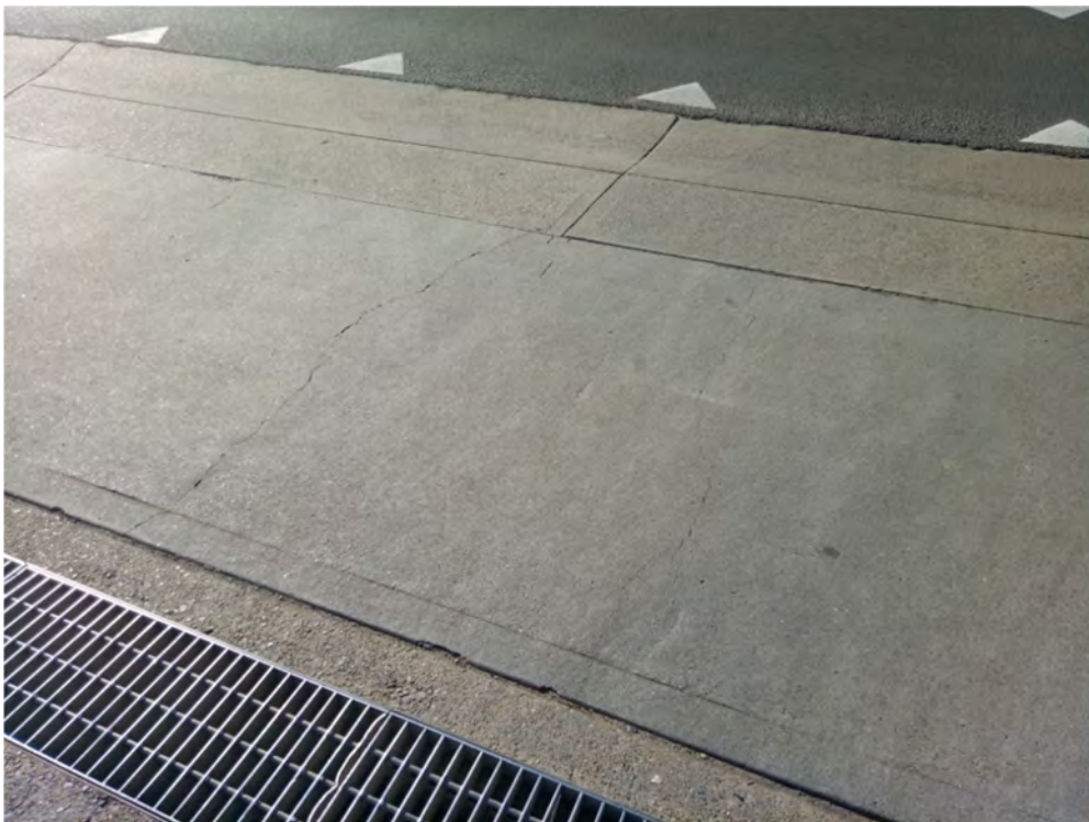
Photo (56): Existing cracks in St Marys manufacturing facilities visitors & staff entry
