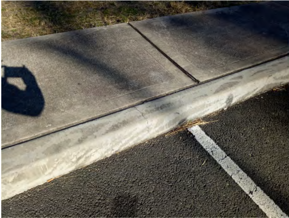
Photo (3): Existing crack in the kerb
