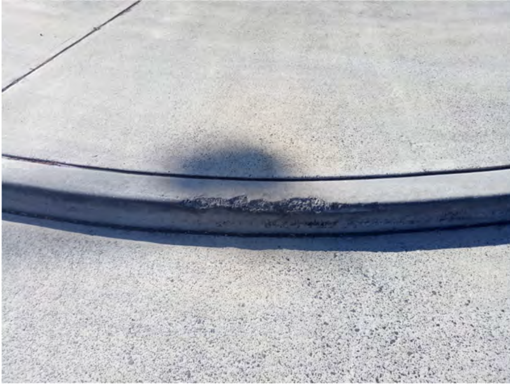
Photo (37): Existing damage in the roundabout
