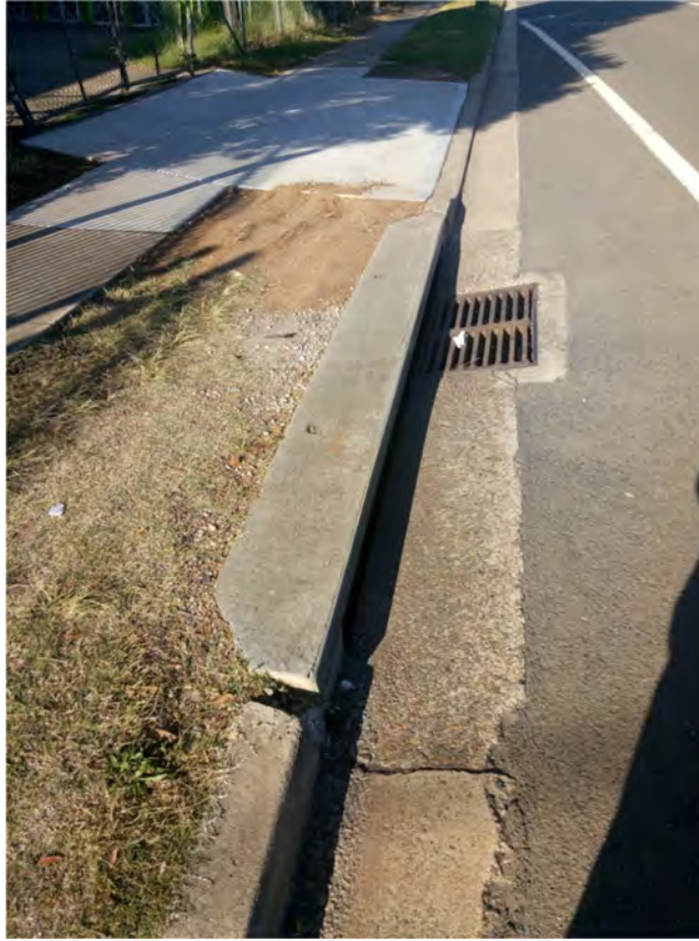
Photo (87): Existing damage in the kerb & gutter along Forrester road (site opposite side)
