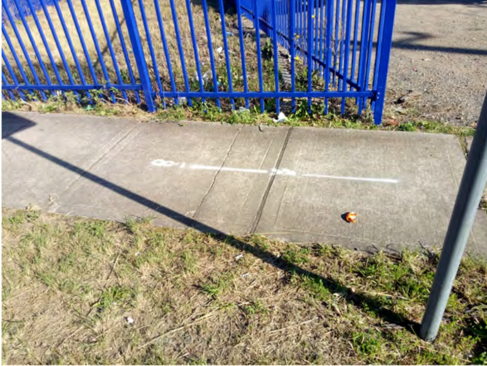
Photo (43): Existing crack in the footpath at the site entry
