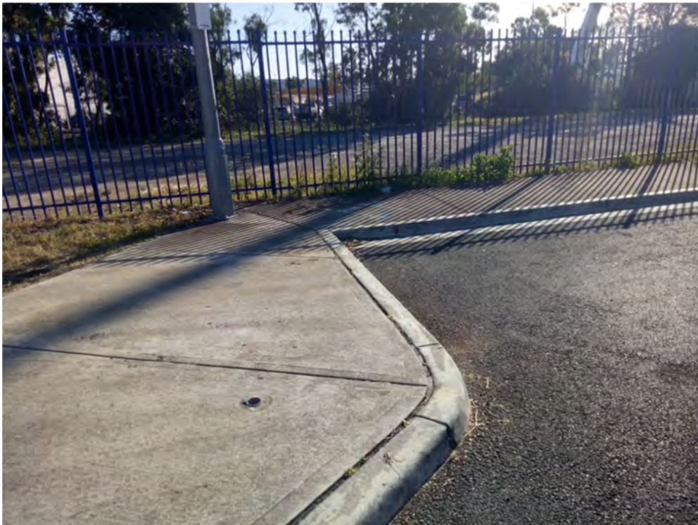
Photo (10): Existing damage in the kerb adjacent to the site
