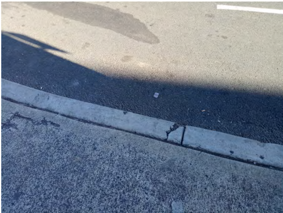
Photo (26): Existing cracks in the kerb at the roundabout area
