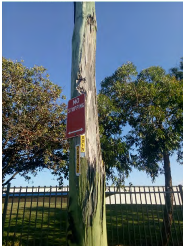
Photo (75): Existing damage in the timber pole along Forrester road (site same side)
