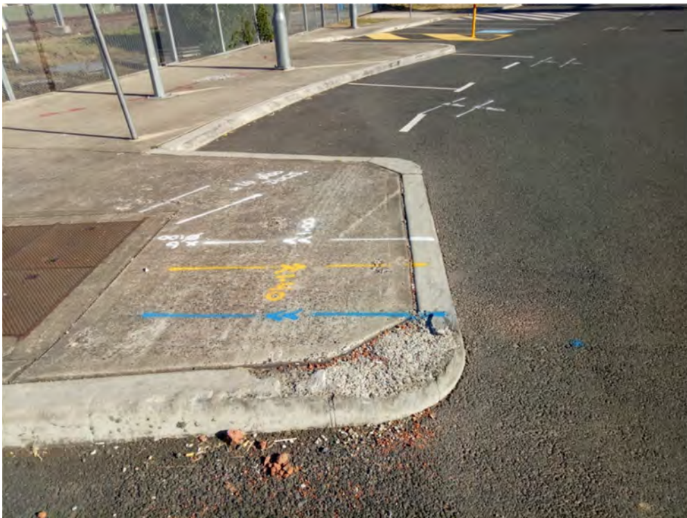
Photo (30): Existing damage in the kerb at the roundabout area
