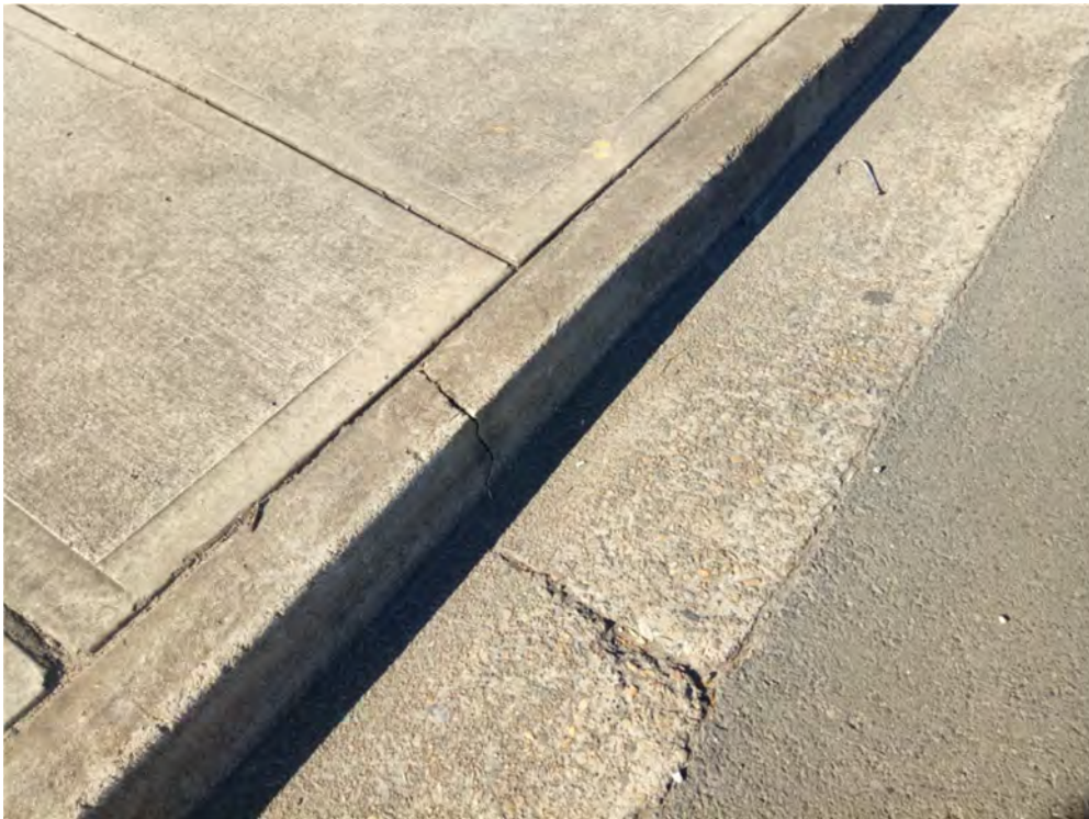
Photo (22): Existing cracks in the kerb & gutter in front of the site entry
