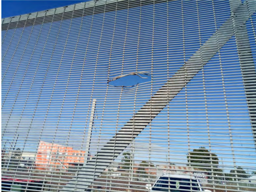
Photo (35): Existing damage in the train station gate at the roundabout area
