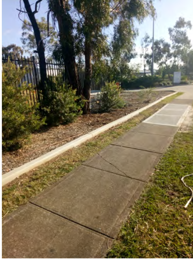
Photo (64): Existing cracks in footpath along Forrester road (site same side)
