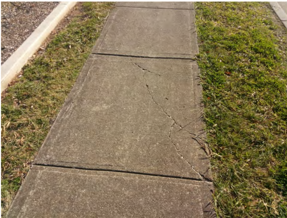
Photo (63): Existing cracks in footpath along Forrester road (site same side)
