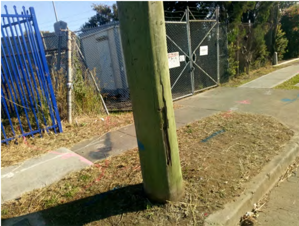
Photo (46): Existing damage in the timber pole at the front of the site entry
