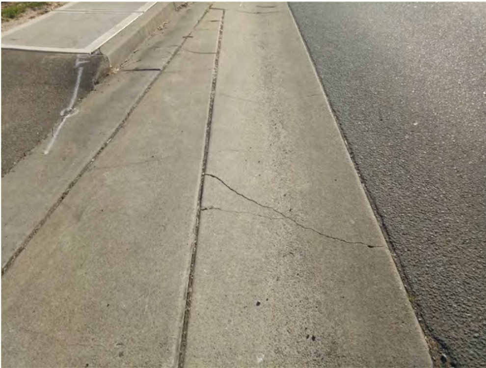
Photo (71): Existing cracks in the gutter along Forrester road (site same side)
