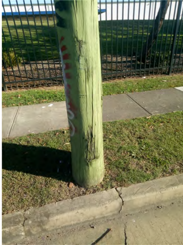
Photo (76): Existing damage in the timber pole, kerb & gutter along Forrester road (site same side)
