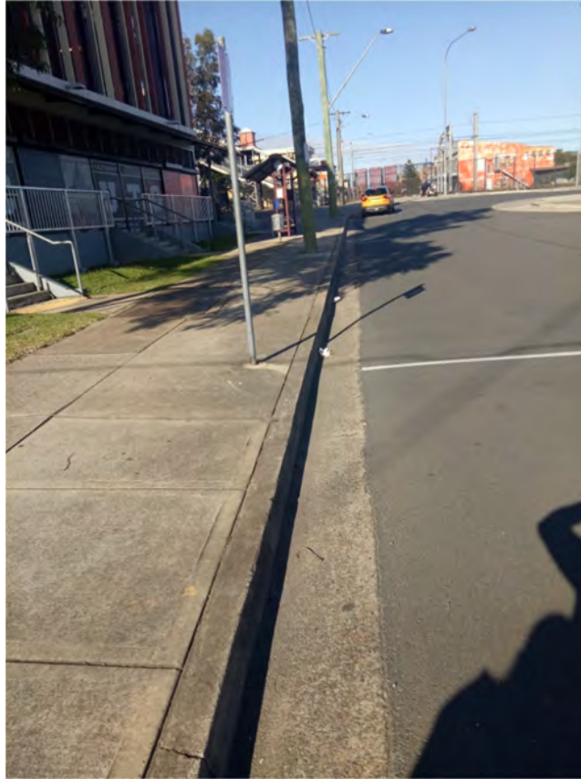
Photo (21): Existing cracks in the kerb & footpath in front of the site entry
