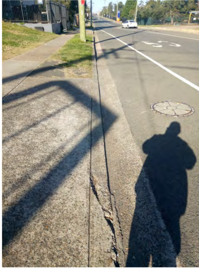
Photo (85): Existing damage in the kerb & gutter along Forrester road (site opposite side)
