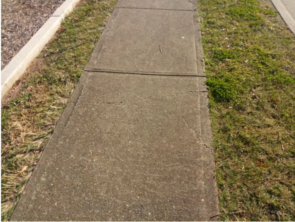
Photo (62): Existing cracks in footpath along Forrester road (site same side)
