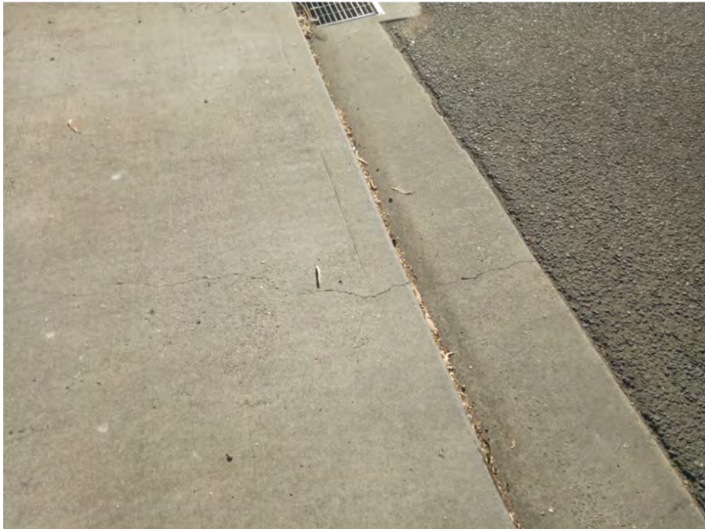
Photo (81): Existing cracks in Stockland entry driveway along Forrester road (site same side)
