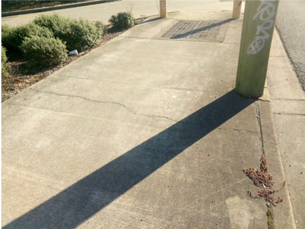
Photo (68): Existing cracks in footpath along Forrester road (site same side)
