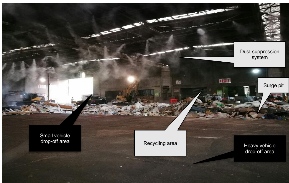
Figure 10: Dust Suppression System in the WTS
