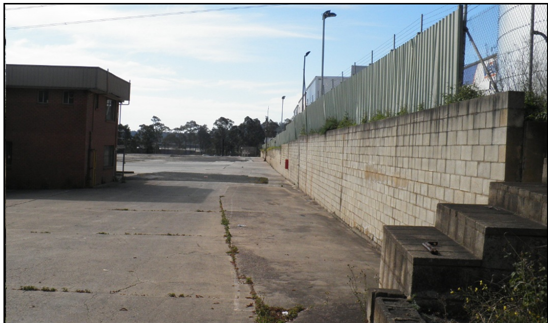
Photograph 10: This photograph shows the existing retaining wall located on the eastern boundary of the Site. The property to the east has been significantly filled behind the retaining wall.
