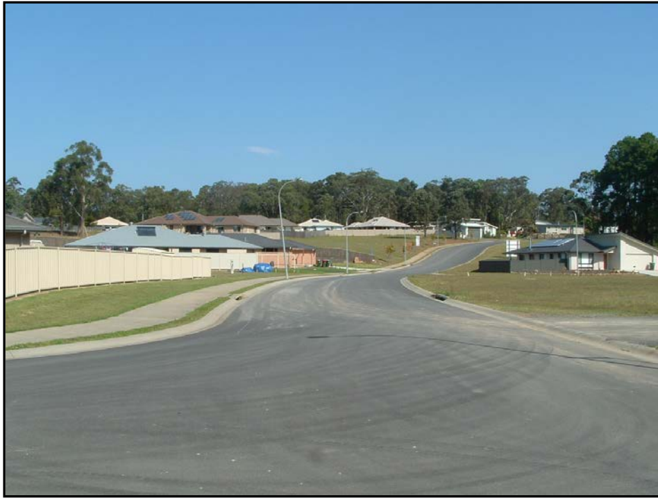
Photo 3 – View along Collector Road showing the cross section. Note off road shared path to left hand side of photo.
