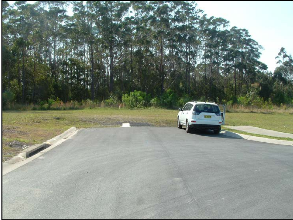
Photo 1 Existing stub on Collector Road (8.0 metres wide) allowing for future access for residential land
