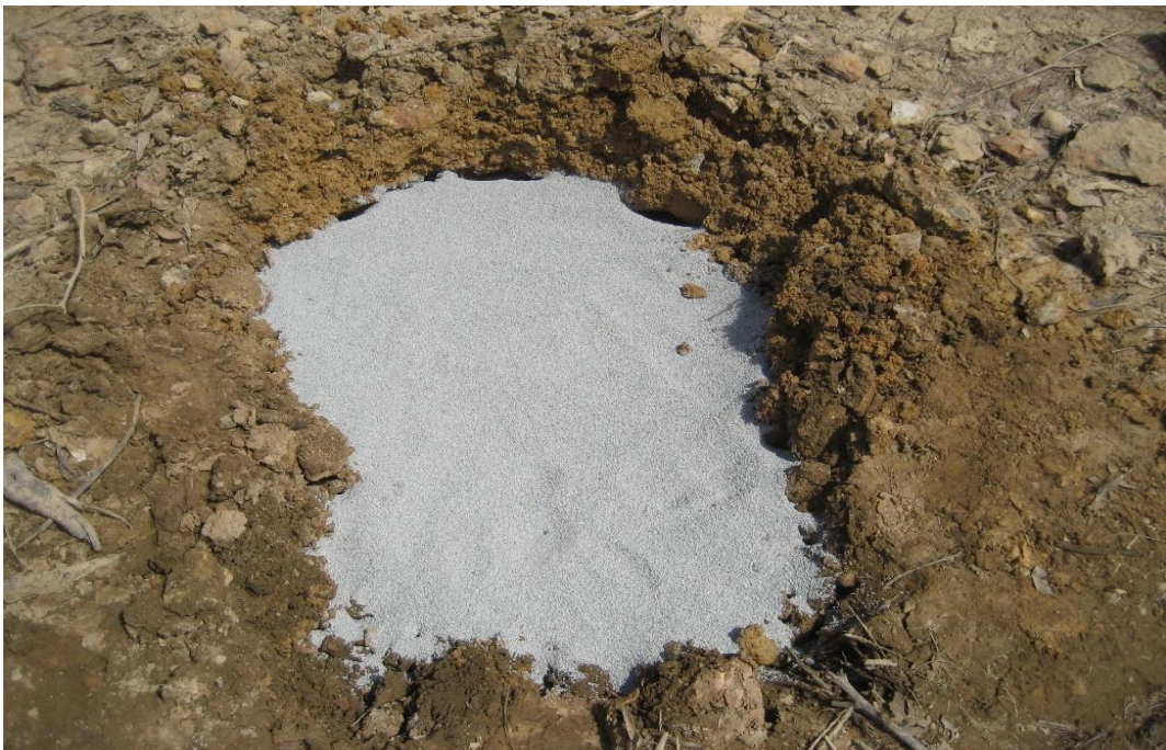
Photo 7: Bentonite used to backfill test pits in leachate dam liner.
