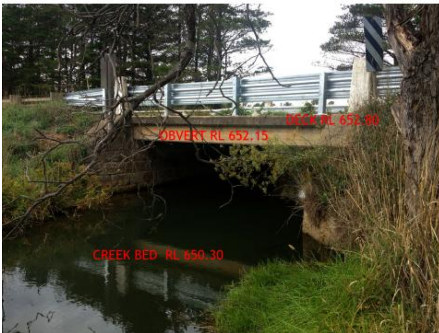
Photo 2 Old Hume Highway plank bridge
