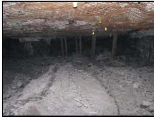
Figure 10. Moderate Floor Heave in 3-North Panel (outbye)
