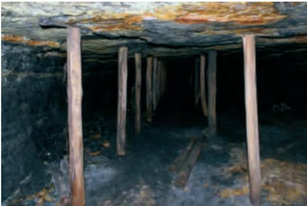
Figure 10 (above): Loch Catherine Colliery underground workings in the Wongawilli Seam, located about 2km north of the Hume Coal project – age of workings is estimated to be 80 years. No obvious rib spall or rubble pile is evident.
