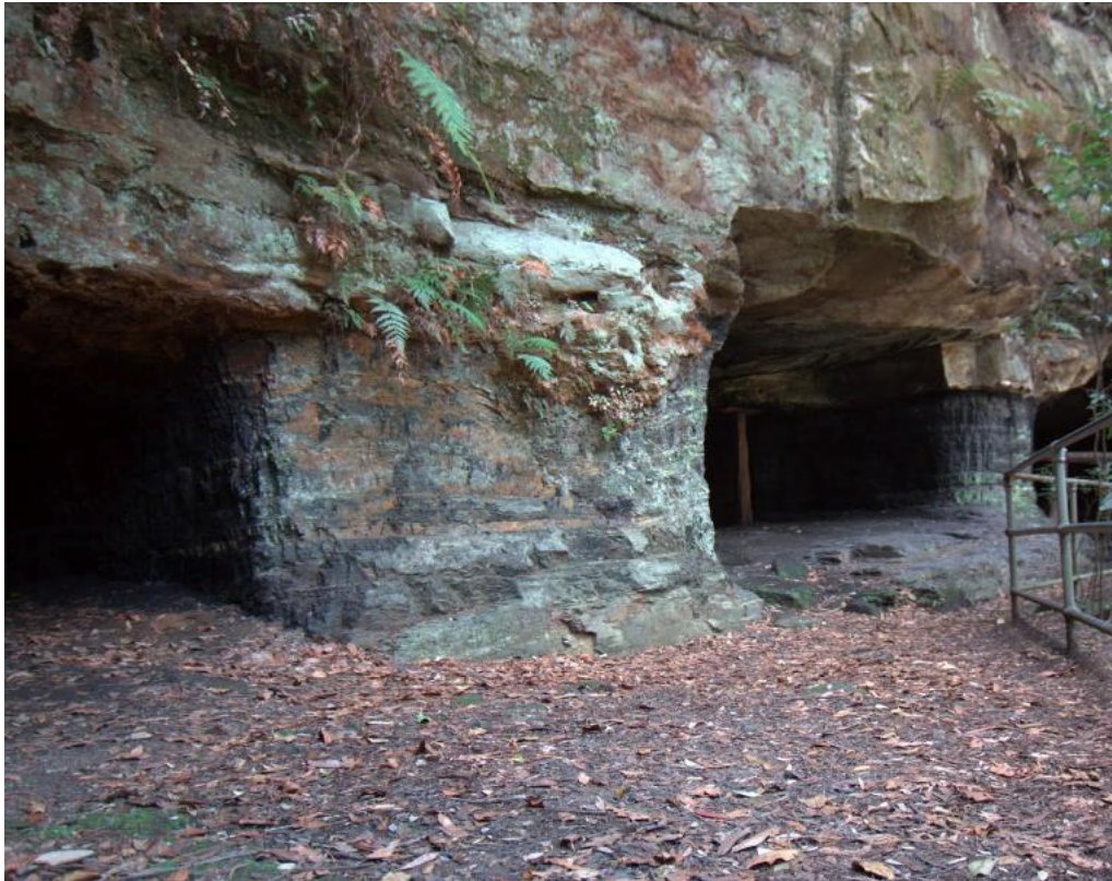
Figure 13(above): Erith Colliery adits in the Wongawilli Seam, located about 8km south of the Hume Coal project – age estimated to be 150 years. No evidence of rib spall.
