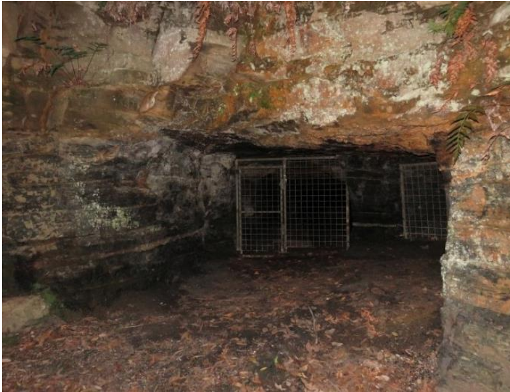
Figure 11 (above): Erith Colliery adit in the Wongawilli Seam, located about 8km south of the Hume Coal project – age estimated to be 150 years. No evidence of rib spall.
