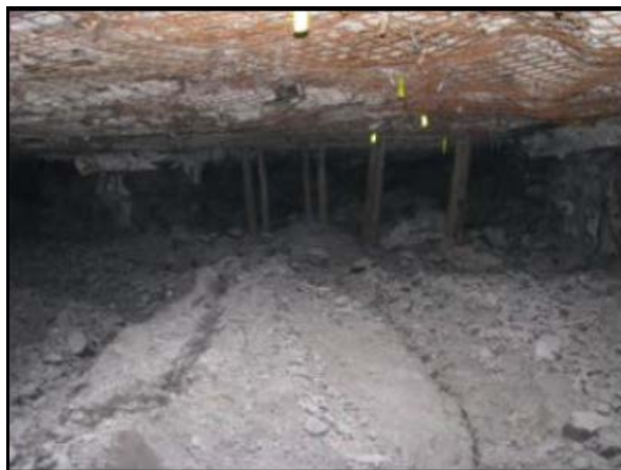
FIGURE 36. Moderate Floor Heave in 3-North Panel (outbye)
