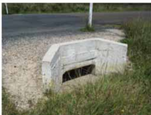
Photo 1.6 Photo of Eastern box culvert looking downstream
