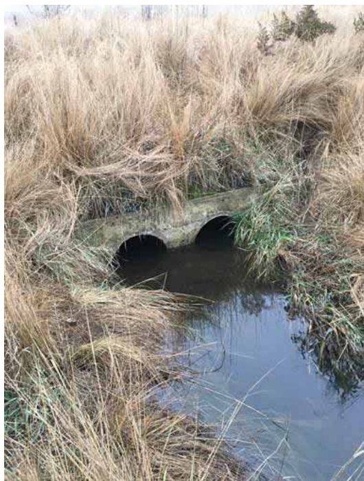
Photo 1.9 Photo of culvert under old rail embankment on eastern side
