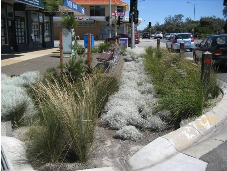
Typical bioretention trench
