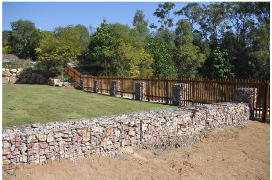
Gabion wall - Signage base
