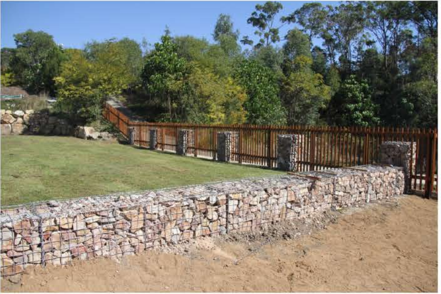
Gabion wall - Signage base
