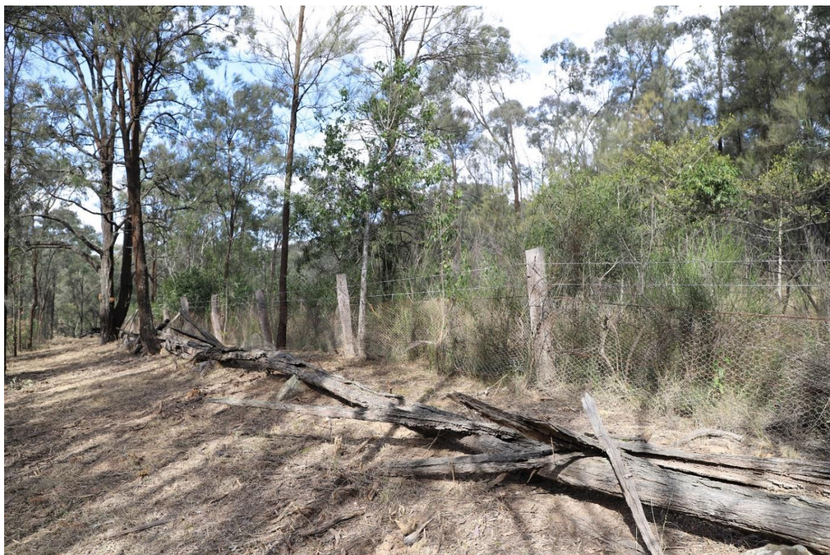
Photo 4.2 Section 2 of the fence, illustrating the deterioration of timber elements
