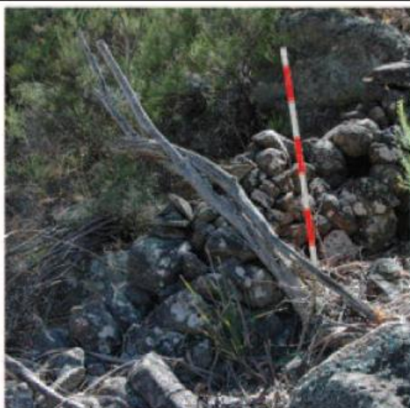
A cut fork resting across the wall still retains the cut pole that was originally supported by dog-legs at its uphill end.
