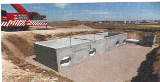
Figure H.13 A treatment chamber constructed out of precast panels (Source: Stormwater360)
