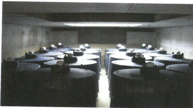
Figure H.11 A fully installed and operational StormFilter system (Source: Stormwater360)
