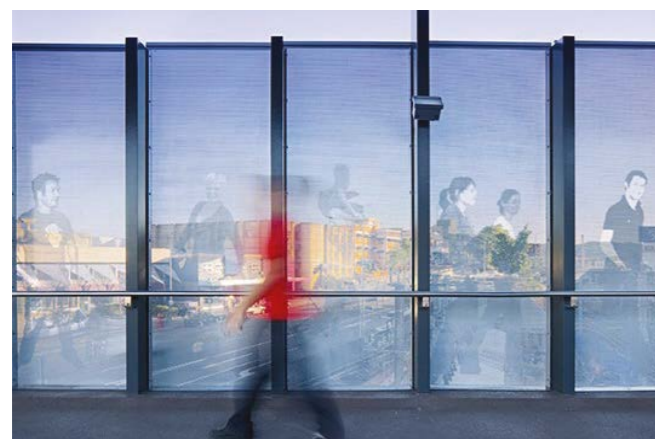
1. Expanded mesh fence - 1800 high
