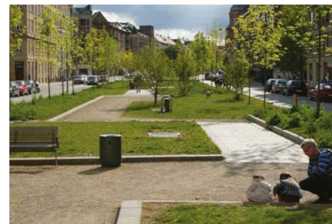
3. Slightly raised turf area with robust edge
