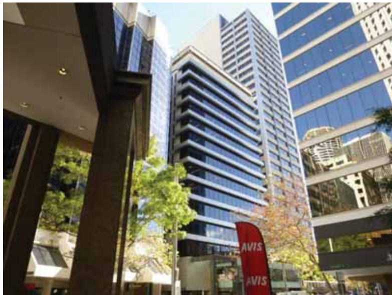
Plate 2: Fairfax Building in the middle of the photo
