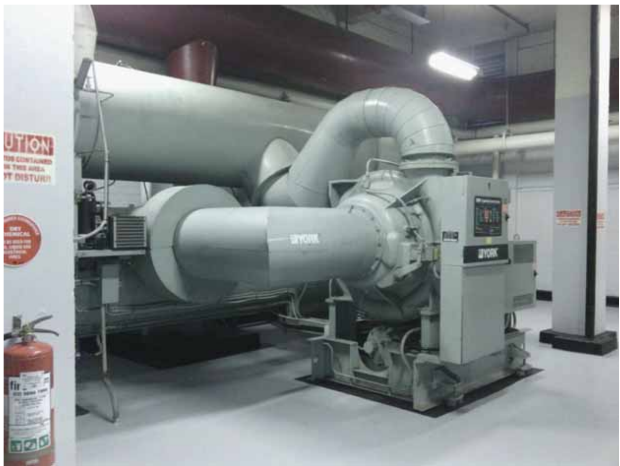
Plate 17: Pumps for Chillers within Level 26 of Goldfields House Building
