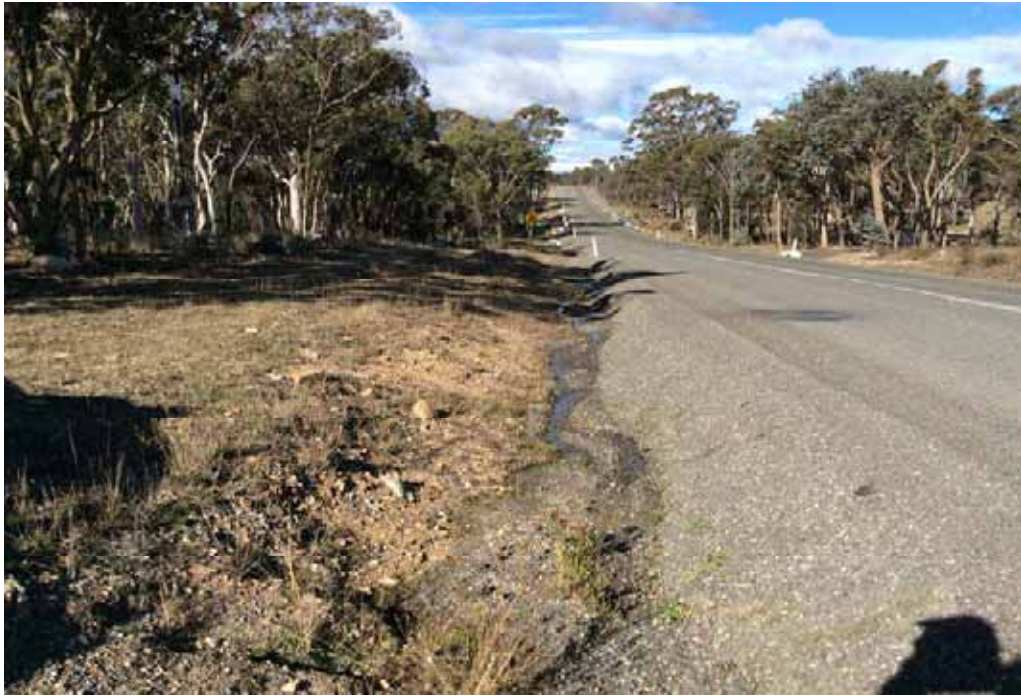
Photo P3 Table drain and batters in clear zone on northern side of Brayton Road. Barrier lines faded. Narrow Road sign in advance of guardrails at road culvert. No edgelines Ch 2.70Km.
