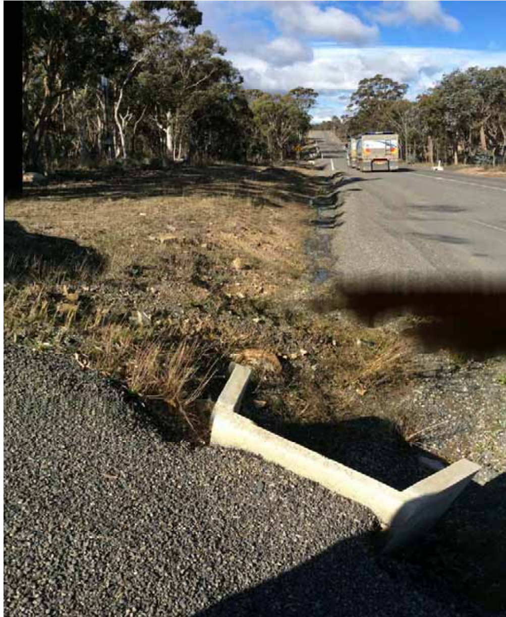
Photo P2: Headwall in pipe crossing at driveway entrance in clear zone on northern side of Brayton Road. Unclear where sealed shoulder joins edge of through lane CH 2.70 Km.
