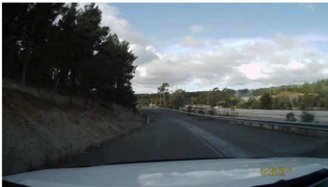
Video Photo V8: View eastbound on Red Hills Road east about 100 metres from Hume Highway tee intersection. Dividing barrier lines BB faded. Hard to see. CH 7.60Km.
