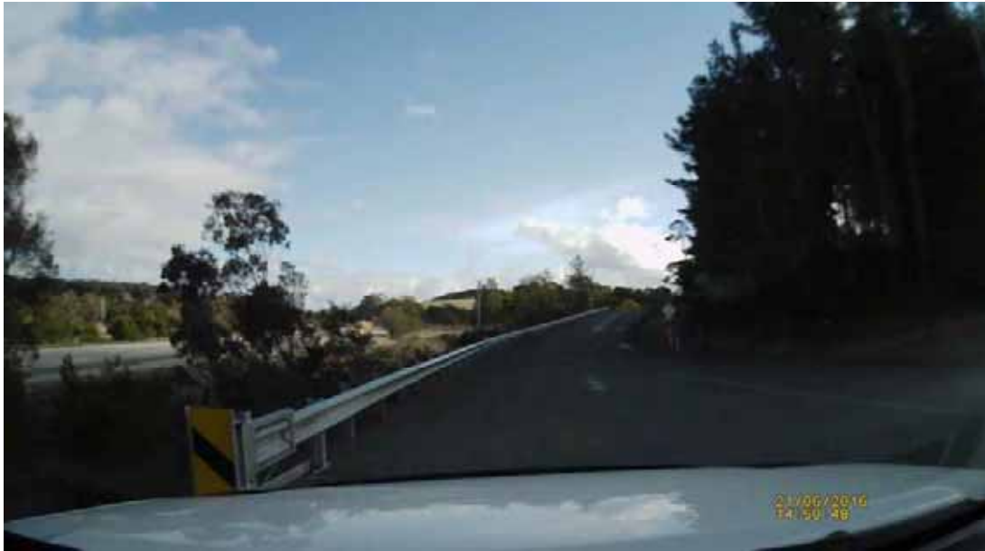
Video Photo V9: Guardrail on left on curve to right and crest ahead. Dividing barrier lines BB faded. Ch 0.10 Km
