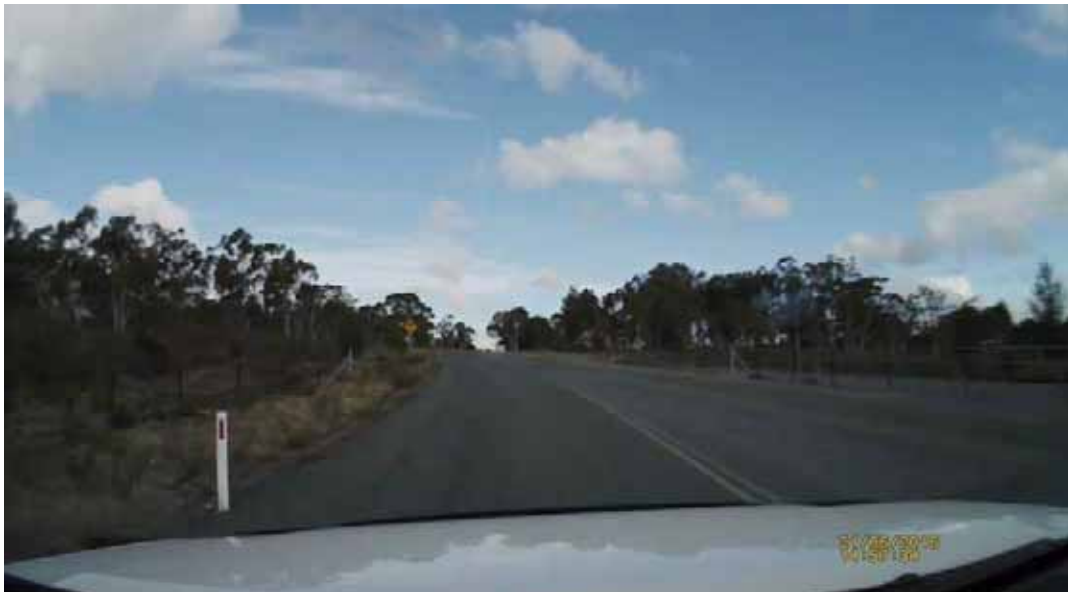
Photograph V10: View westbound on Brayton Road about 100 metres west of tee intersection with Bypass Road. School bus route sign on left. Dividing barrier lines BB (two way) faded. Ch 3.60 Km
