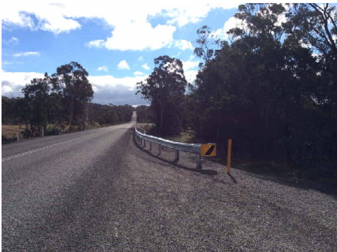
PHOTO P1 View west of Brayton Road from bus stop on northern side. Unclear where edge of shoulder seal joins edge of through lane.
