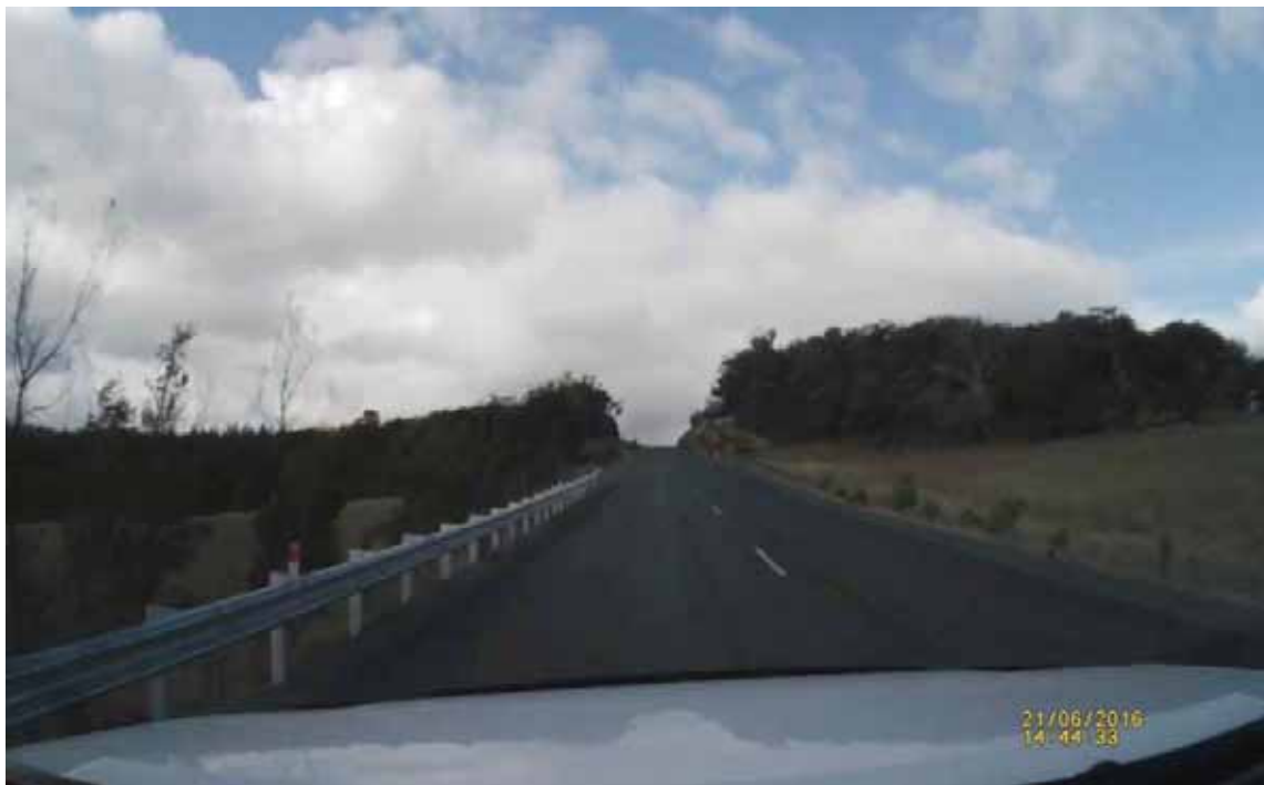
Video Photo V6: Dividing separation line S1 on steep 12% gradient in Bypass Road eastbound. Guardrail on left. Steep drop off CH 5.75 Km.
