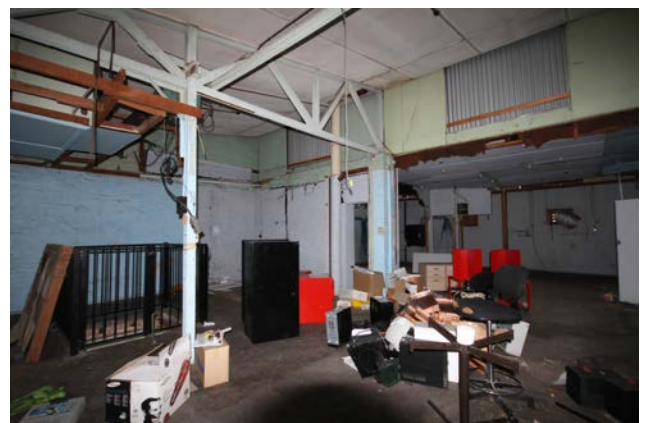
Figure 3.24 First floor view, showing original timber roof trusses
