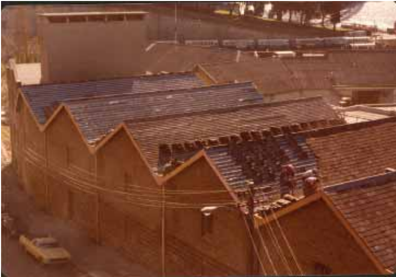
Figure 2.23 c.1970s Campbell's Stores at the time of re-roofing with slate. Note the masonry chimney/vent between Bays 10 and 11 to the upper left
