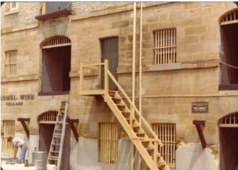
Figure 2.24 c.1970s Eastern facade of Campbell's Stores with areas of render to the ground floor level before remediation. Note the original location of the stairs to the first floor level, reflecting the original tenancy separation of each floor
