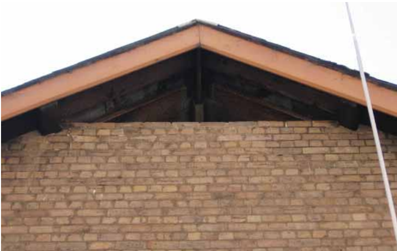
Figure 2.33 left Hickson Road elevation detail of Bay 7 of Campbell's Stores showing the gable vent without the installation of a louvre (refer Figure 5.7)
