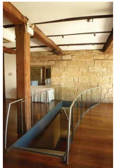
Figure 3.15 An example of a contemporary stair inserted between the column grid (Bay 5). Note the brickwork to the top of the sandstone and the infill below the beams where the former roof structure was bearing
