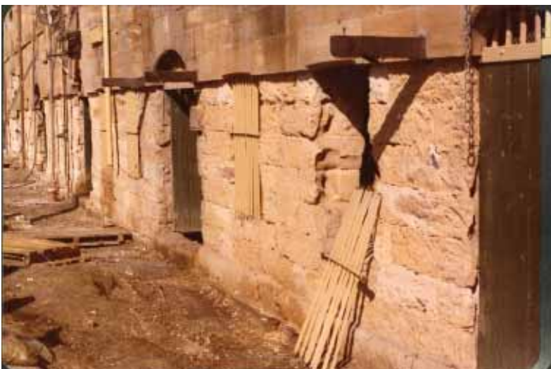
Figure 2.25 c.1970s Campbell's Stores after the removal of the weathered sandstone and before replacement, to the ground floor level of the eastern facade
