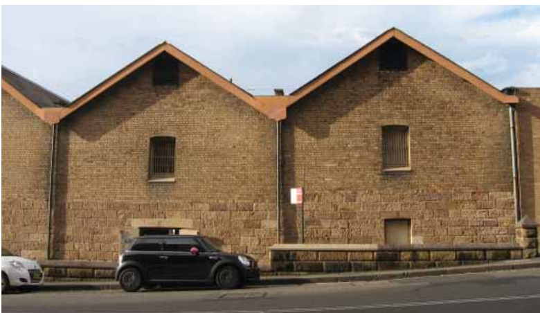
Figure 5.6 left Hickson Road elevation (west) of the subject building with Bays 1 and 2. Note the vent openings to the gable apex, proposed to be altered
