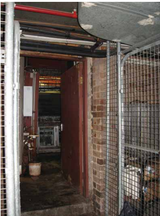
Figure 3.14 Services tunnel below the Hickson Road footpath, with a doorway to the building on the left, the original sandstone wall between the door frame and the brickwork skin next to it on the right
