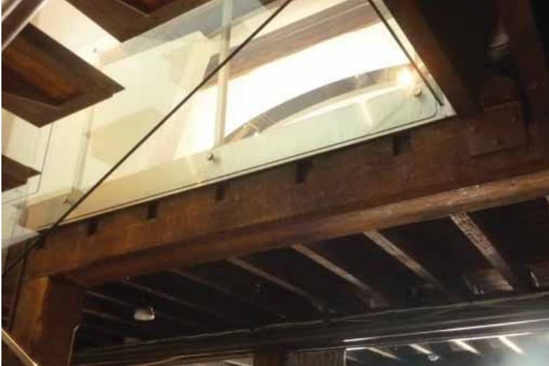
Figure 3.12 A contemporary stair opening showing the main beam structure with floor joists to one side and the notched recesses where the joists have been removed (Bay 2)
