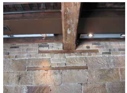
Figure 2.9 Second level wall indicating a main beam for the third level floor that was added c.1885, and its raised position relative to the position of the original roof beam 'pocket' with brick infill, to its lower left. Note the change from stonework to brickwork with the third level addition
