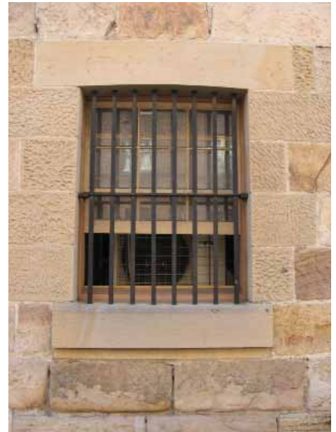
Figure 3.20 Hickson Road window with an A/C unit using the open window for ventilation
