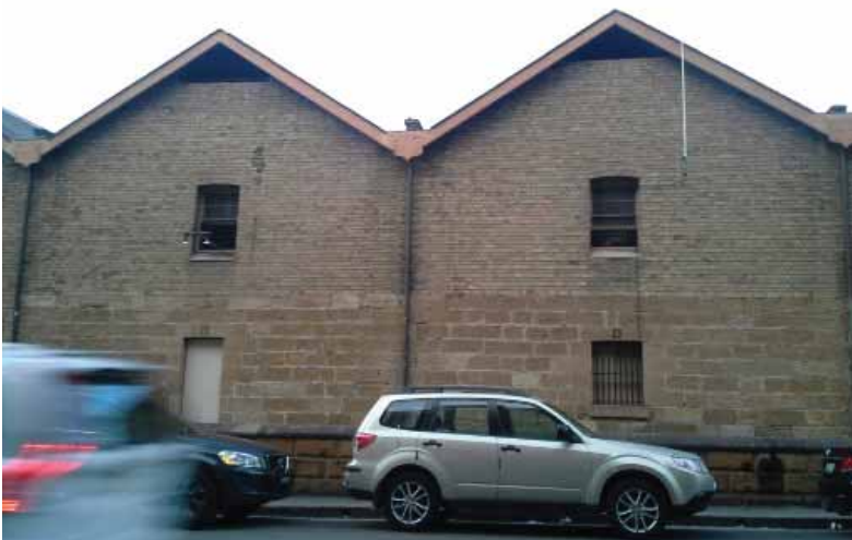
Figure 5.7 Hickson Road elevation (west) of the subject building with Bays 7 and 8 and the 2005 vent openings to the gable apex, but without any louvres. These vent openings are proposed for all the gable ends to achieve ventilation requirements.
