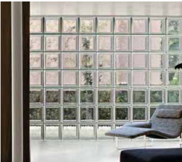
MATERIALITY: The building is intended to be as transparent as possible in order to contrast the existing stores building. Glass blocks are proposed to address acoustic, thermal and visual issues such as the privacy of residents at No. 8 Hickson Road and the Park Park Hyatt.
