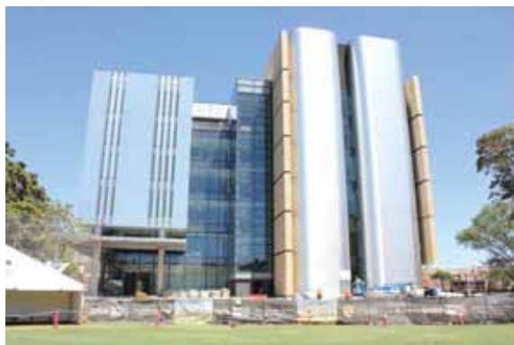
Figure 3.11 Charles Perkins Centre, under construction. (Source: GML 2013)
