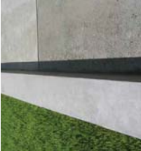
W2 - CUSTOM WALLS - IN-SITU CONCRETE RETAINING WALL
