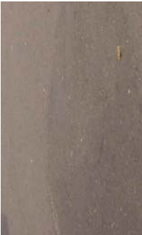
P7 - ASPHALTIC CONCRETE SURFACES
