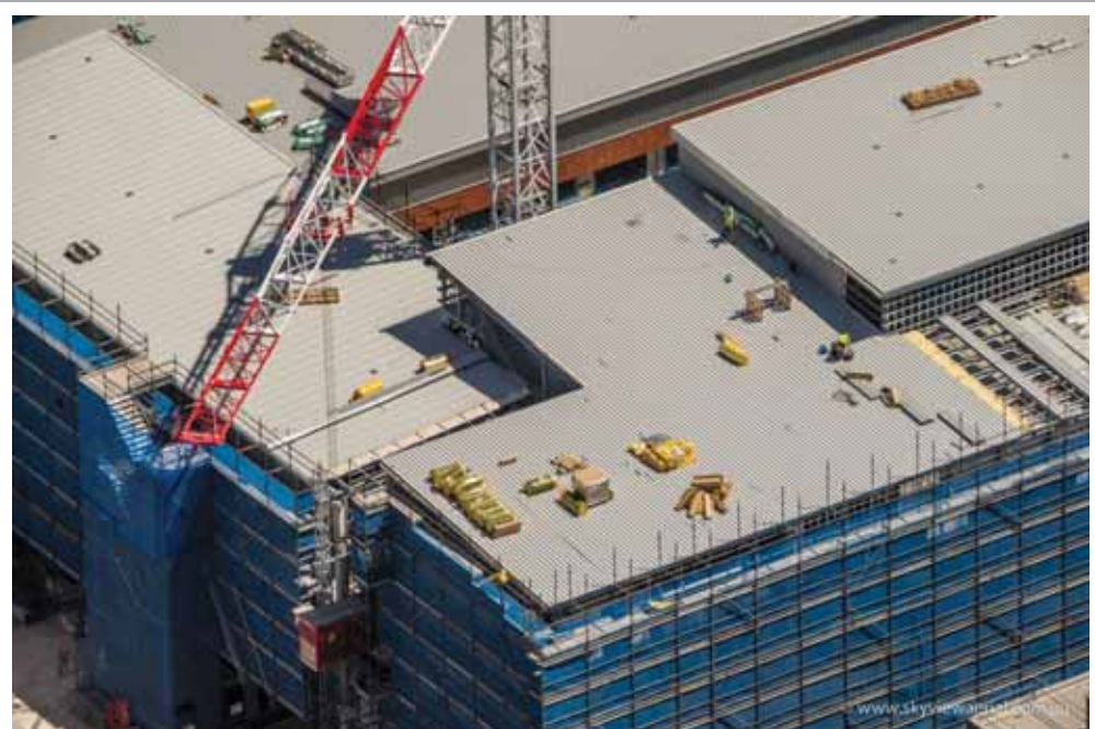
Hornsby Hospital – Internally located tower crane & Externally mounted man / material hoist (both serviced from
