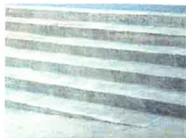
S3 - INSITU REINFORCED CONCRETE STAIR
