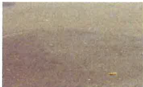
P7 - ASPHALTIC CONCRETE SURFACES
