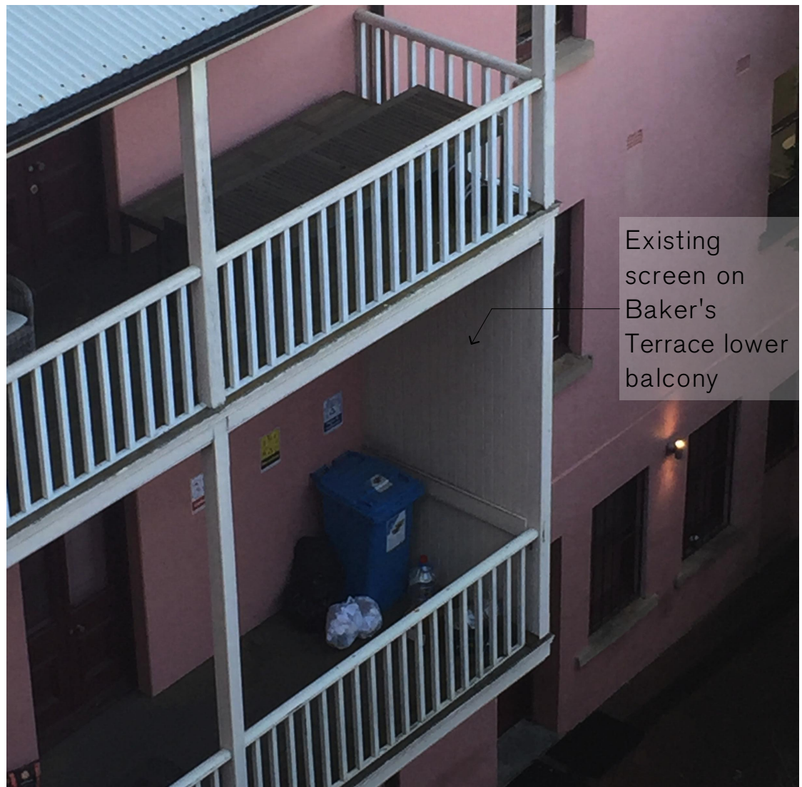
2 Existing Baker's Terrace balcony screen (Level 2)
