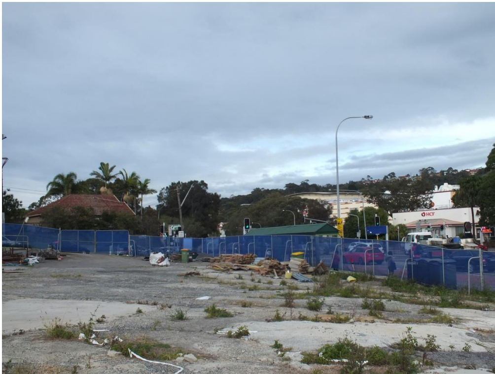
Figure 6.1 View south-west, from near the boundary between 612 & 620 Pittwater Road, showing the remains of the concrete forecourt of the service station, areas of disturbance caused by remediation activities, the storage of some building materials and partial regrowth of grass and weeds in patches.
