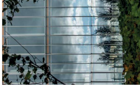
Glass Facade of the shard, London
