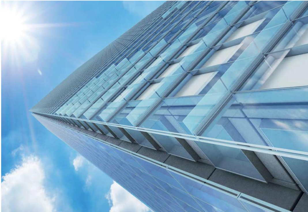
One Sydney Harbour Facade at Notch
