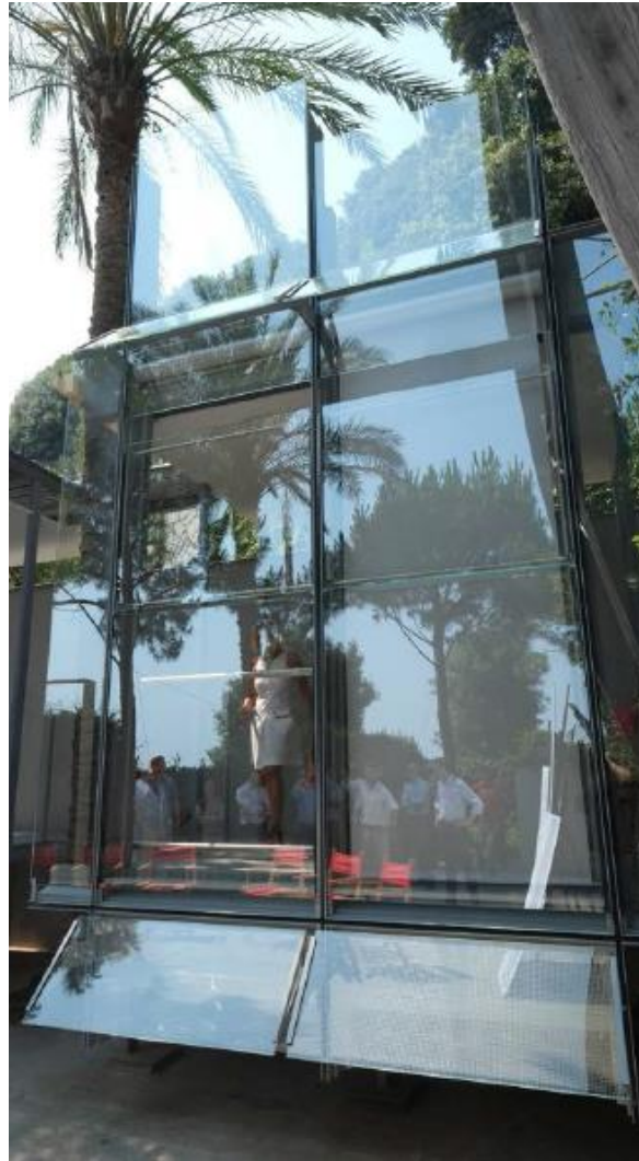
Figure 7 – A full-scale mock-up of the Wintergarden facade
