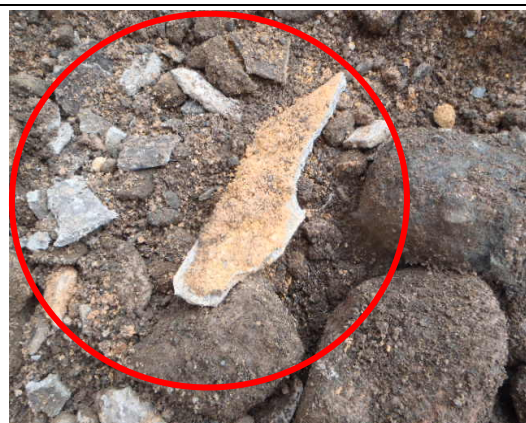
Photo 6. Stockpile 225, Excavation Area – Presumed asbestos-containing fibre cement fragments
