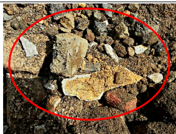
Photo 9. Stockpile 225, Excavation Area – Presumed asbestos-containing fibre cement fragments
