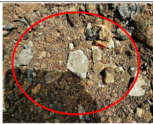
Photo 8. Stockpile 225, Excavation Area – Presumed asbestos-containing fibre cement fragments
