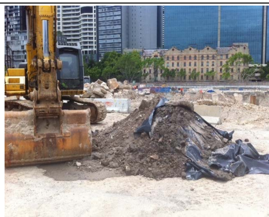
Photo 20. Overview of Stockpile 225, Within C3 exclusion zone
