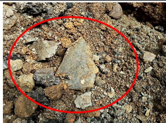
Photo 11. Stockpile 225, Excavation Area – Presumed asbestos-containing fibre cement fragments
