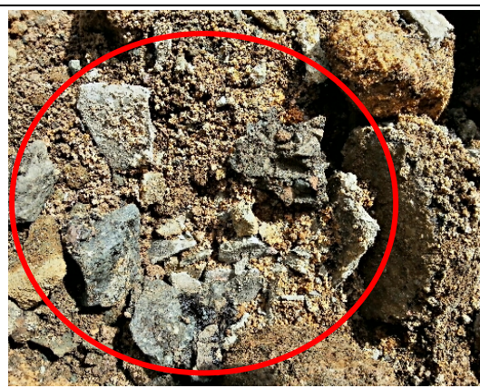
Photo 10. Stockpile 225, Excavation Area – Presumed asbestos-containing fibre cement fragments
