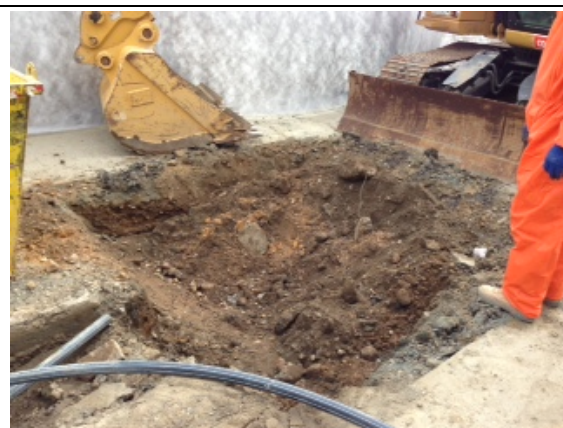
Photo 19. New Amenities Area, Excavation Area, During excavation works
