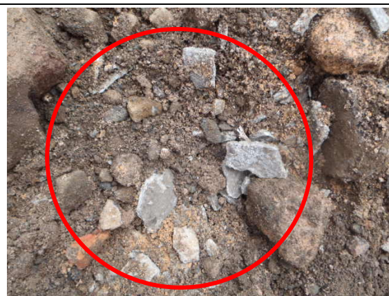
Photo 7. Stockpile 225, Excavation Area – Presumed asbestos-containing fibre cement fragments
