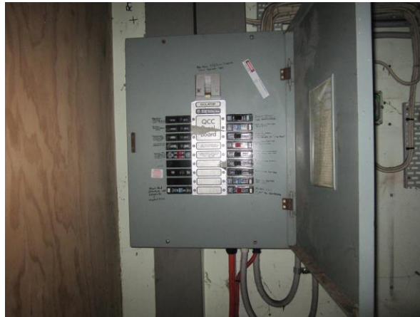
Photo 15: Rear ecx 004, electrical distribution board
