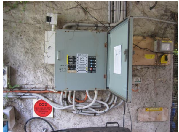
Photo 2: Tapir, electrical distribution board
