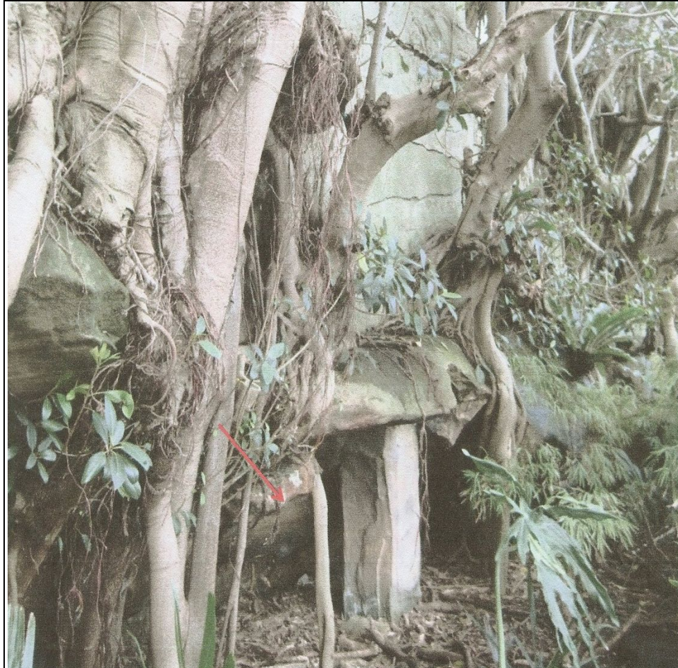
Figure 1.10: This image shows the rock overhang, masonry pillar and several fig trees growing into the rock face. The Aboriginal heritage site (arrowed) is under the overhang to the left of the pillar. A masonry wall is built over the rock overhang which has a masonry pier supporting it (may not actually provide much support).
