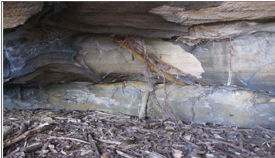
Figure 2.4: The site was inspected again with this photo and the probable location of the photo was identified below and this area of the stone surface below the tree roots is deteriorated here
