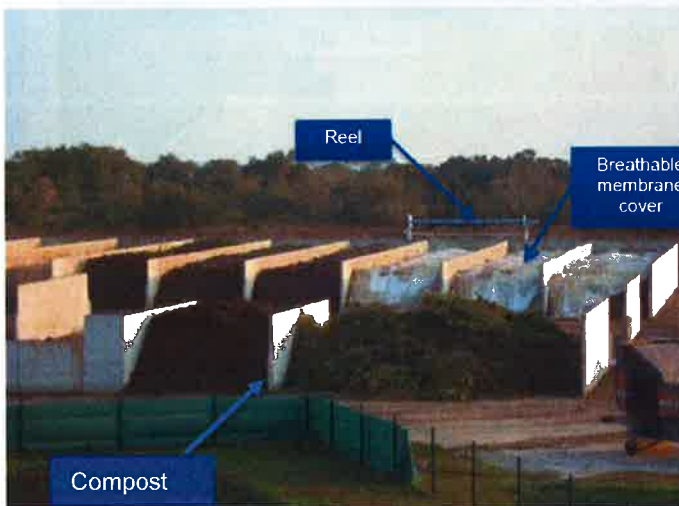
Figure 6: Example of Concrete Bunkers for Composting at GO Facility
