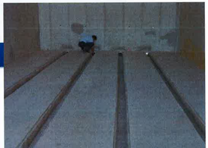
Figure 7: Example of Aerated Concrete Bunker Floor at GO Facility
