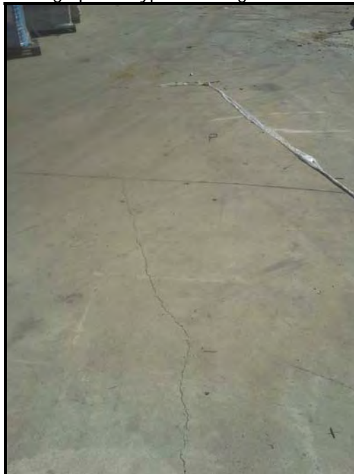
Photograph 2 – Typical Damage to Pavement
