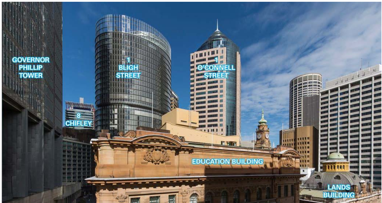
Figure 5: View look south west showing roof of the Education and Lands Buildings and surrounding buildings to the south
