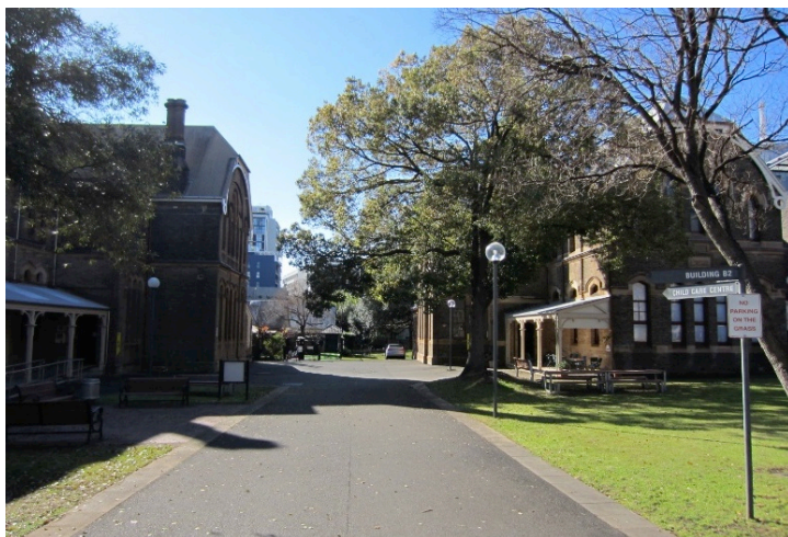
Figure 9. Looking north along the centre of the site between CB22 (left) and CB25 (right) towards the proposed envelope location
