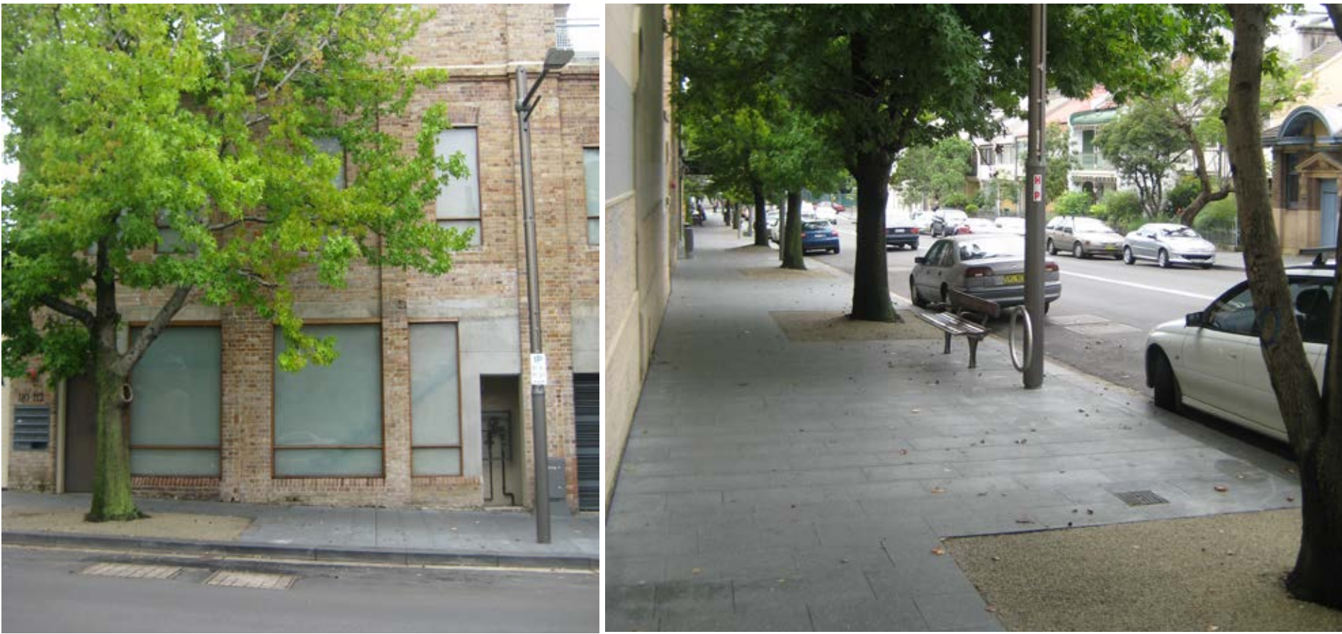
Concrete unit pavement / footpath
