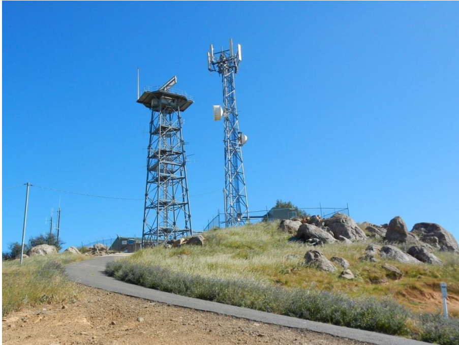
Figure 1 - Mt Bobbara Radar (L) with adjacent mobile tower (R)
